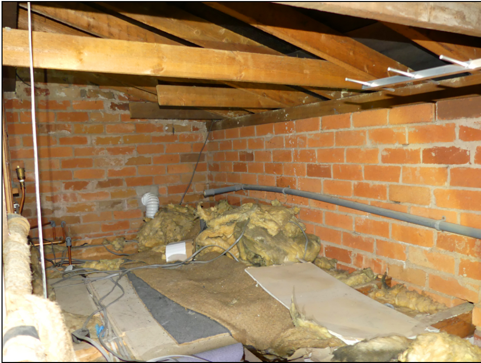
Internal view of roof void, showing internal walls and insulation. February 2020.
