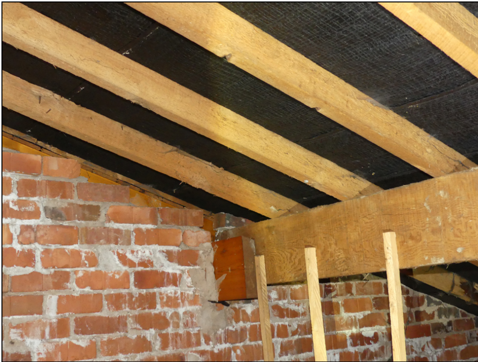
Internal view of roof void, showing roof supports and felt underlining. February 2020.
