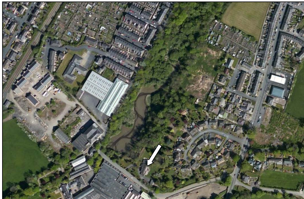
Image 1 – Wide aerial view of proposed development site (marked with white arrow) showing context
