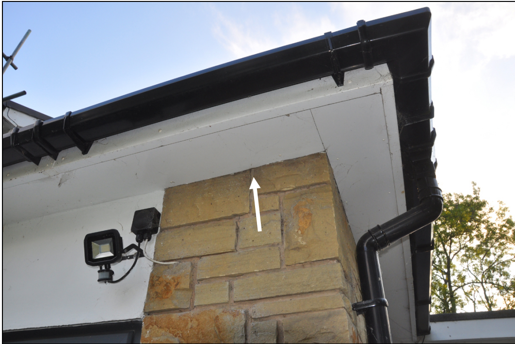
External view of north part of building. Bat emergence point marked by white arrow. May 2020
