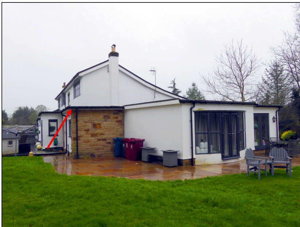
View of Mearley Lodge from north. Bat emergence point marked by red arrow. Image from February 2020.
