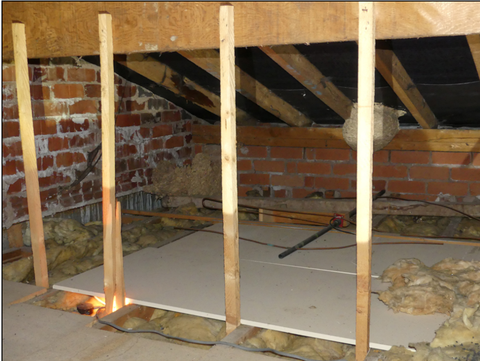
Internal view of roof void, showing roof supports and partial boarding. February 2020.
