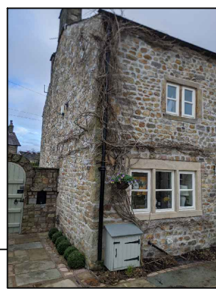
Existing cast rain water goods to the property
