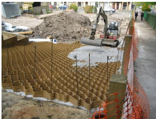
Appropriate aggregates are back filled filling all the cells.
