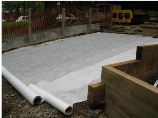
Laying of geotextile fabric with the cellular confinement system pinned in place.
