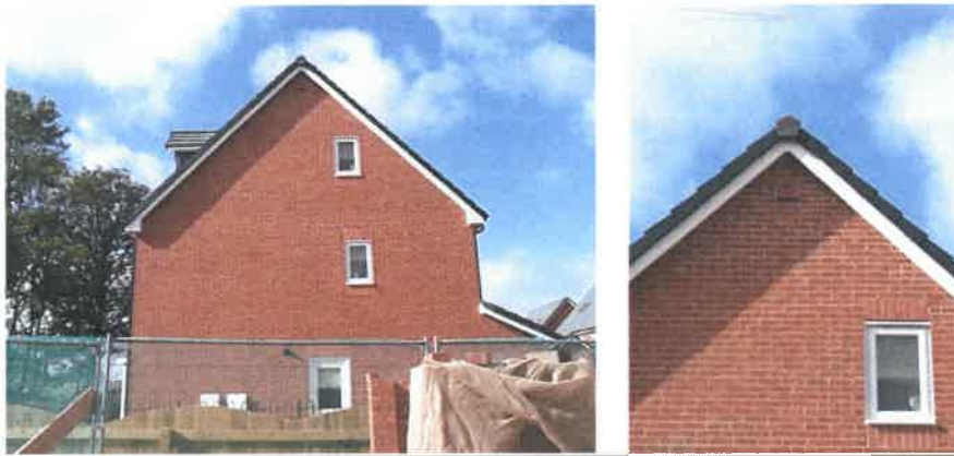
Above: typical unit in situ. Photo © Angela Graham
