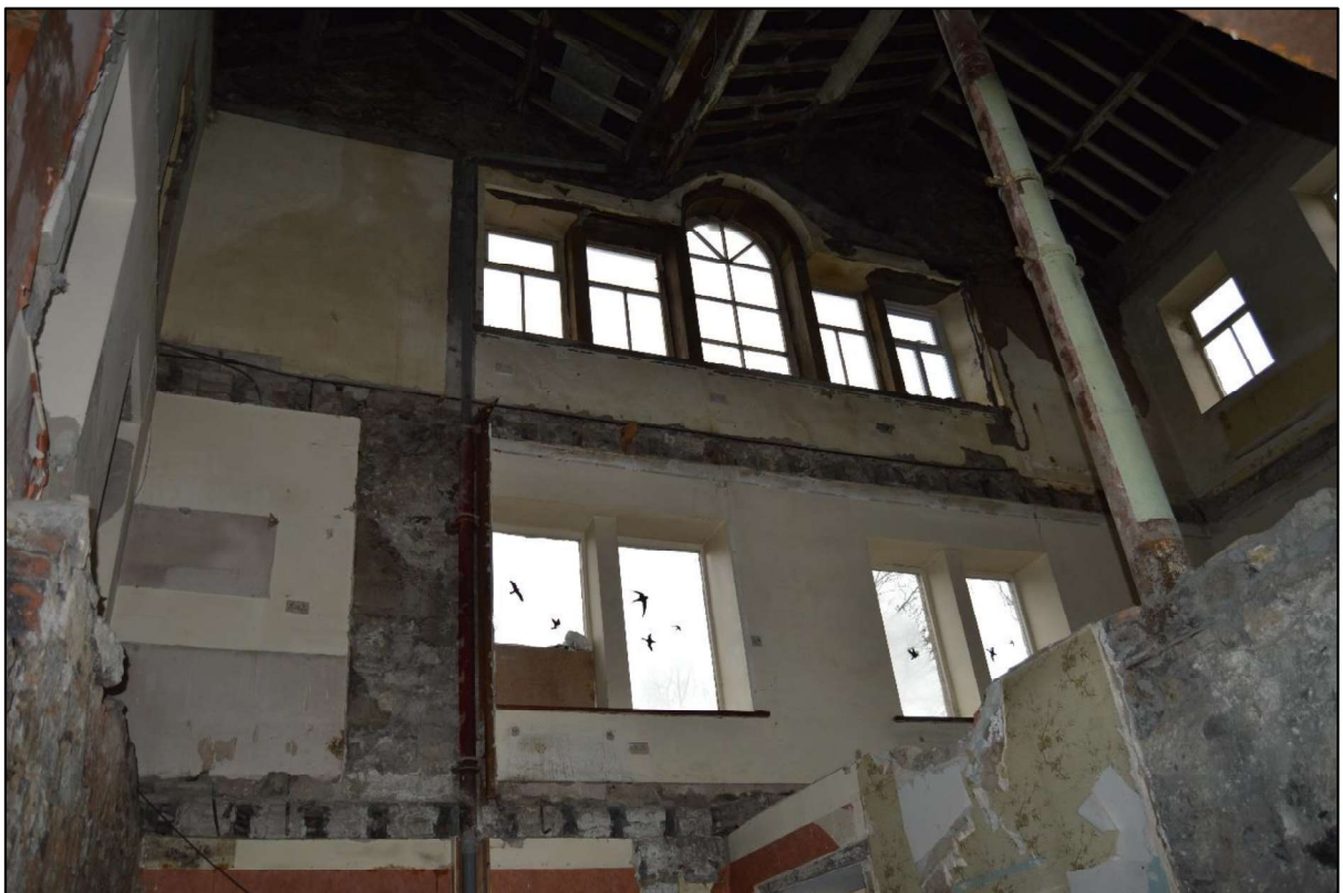
Photo 52: View north east towards the upper levels of the north east gable end of the south range from lower ground floor level.
