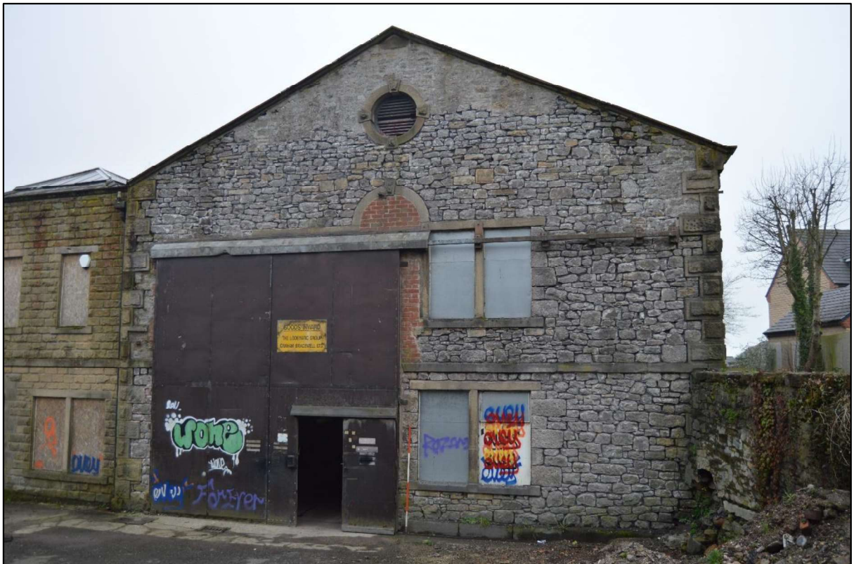
Photo 06: View of the north east gable end to the north range.
