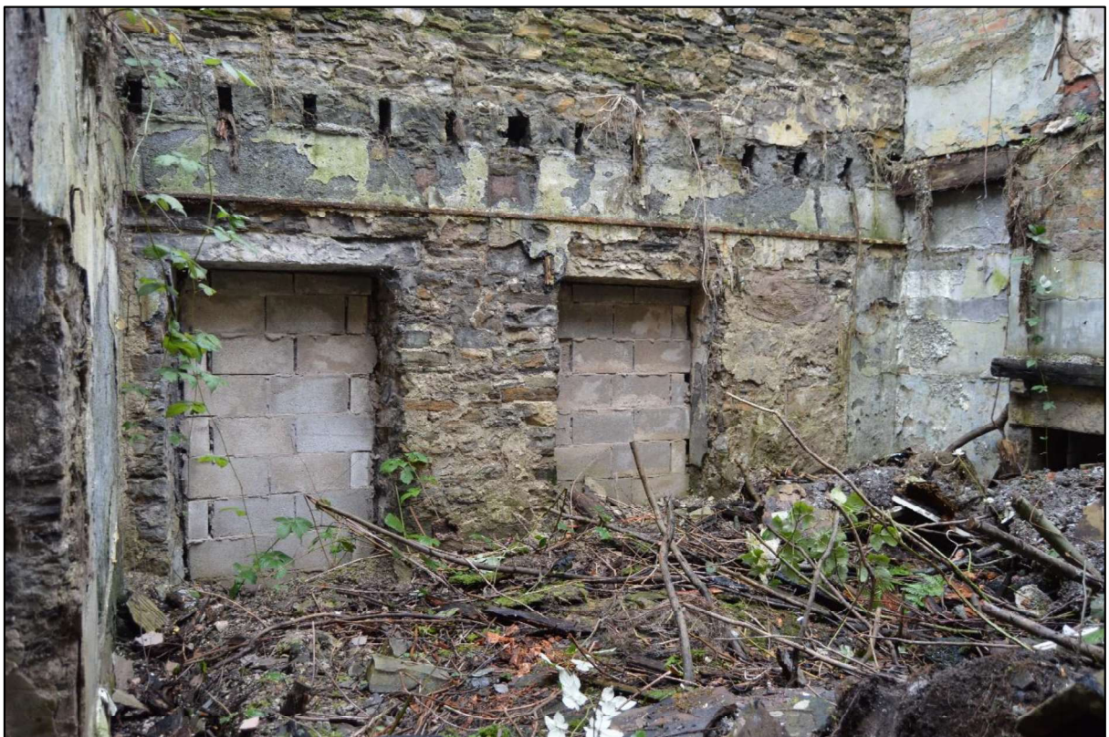
Photo 78: View south west at ground floor level within the south unit of the former cottage.
