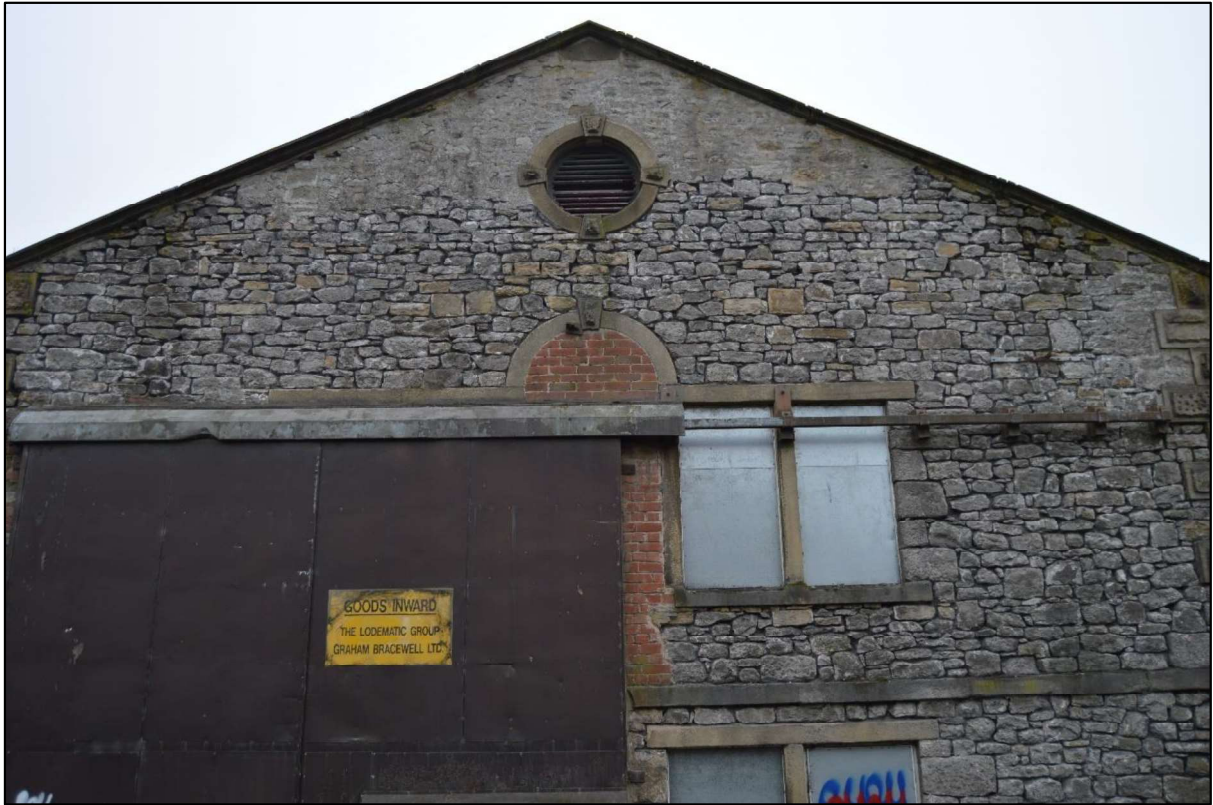
Photo 07: View of the now altered five-light window to the north east gable end of the north range.
