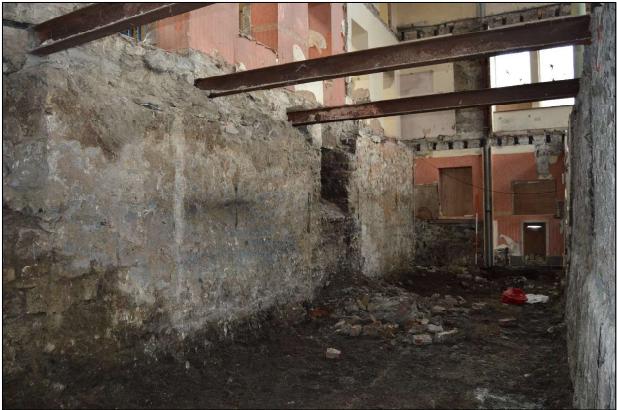
Photo 51: View north along the north section of the south range at lower ground floor level.
