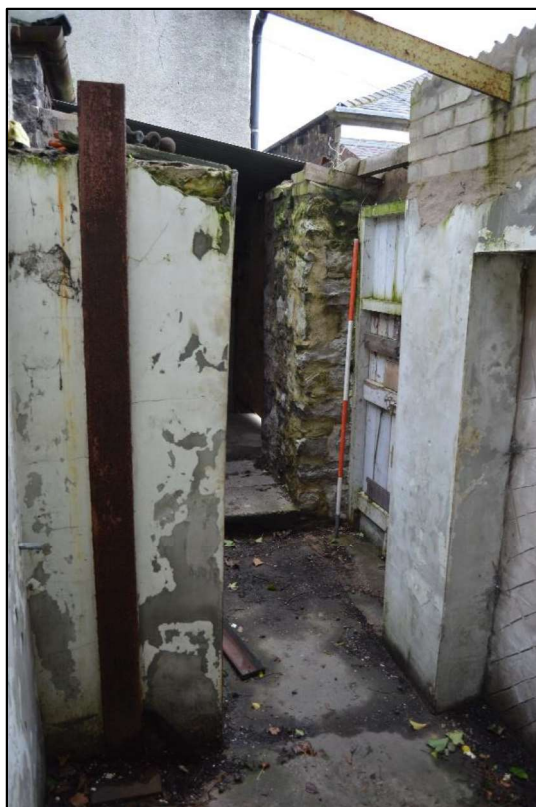
Photo 93: View north east from within the former WC of the south west outbuilding.
