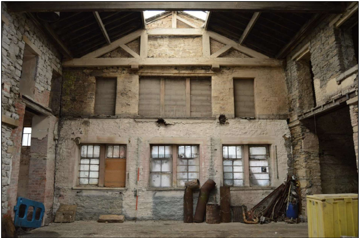
Photo 59: View of the south west gable end of the central range.
