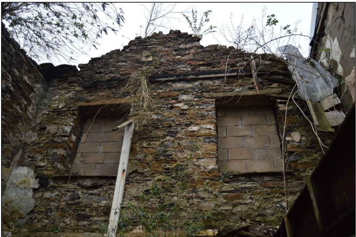
Photo 86: View north west towards the first-floor level of the north west gable of the north unit of the former cottage.
