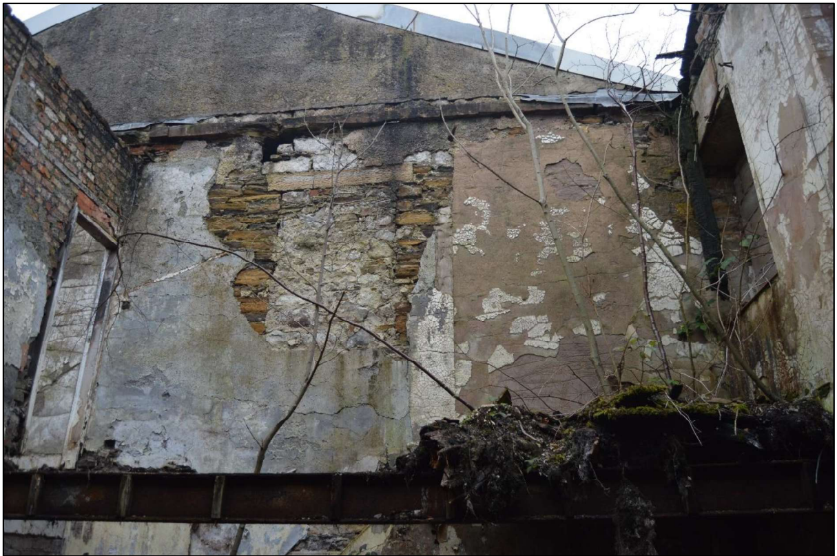
Photo 81: View north east towards the south west gable of the north range from ground floor level within the south unit of the former cottage.
