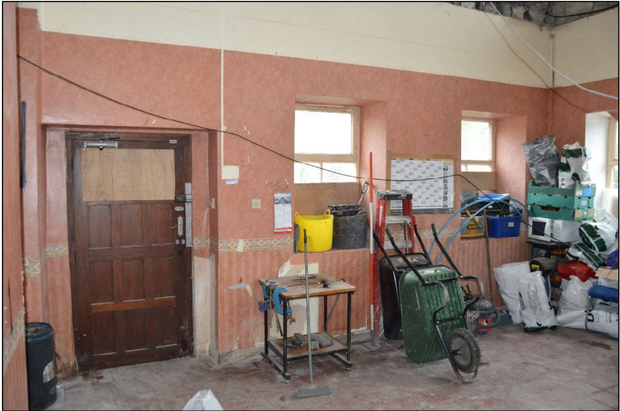
Photo 39: View north east within the north east unit at lower ground floor level to the south range.
