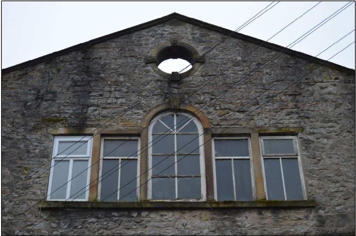
Photo 03: View of the 5-light window with central rounded arched head to the north east gable end of the south range.
