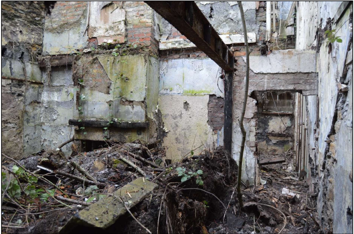
Photo 79: View north west at ground floor level within the south unit of the former cottage.
