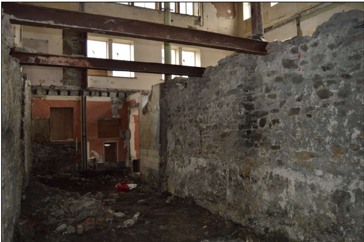
Photo 50: View east along the north section of the south range at lower ground floor level.
