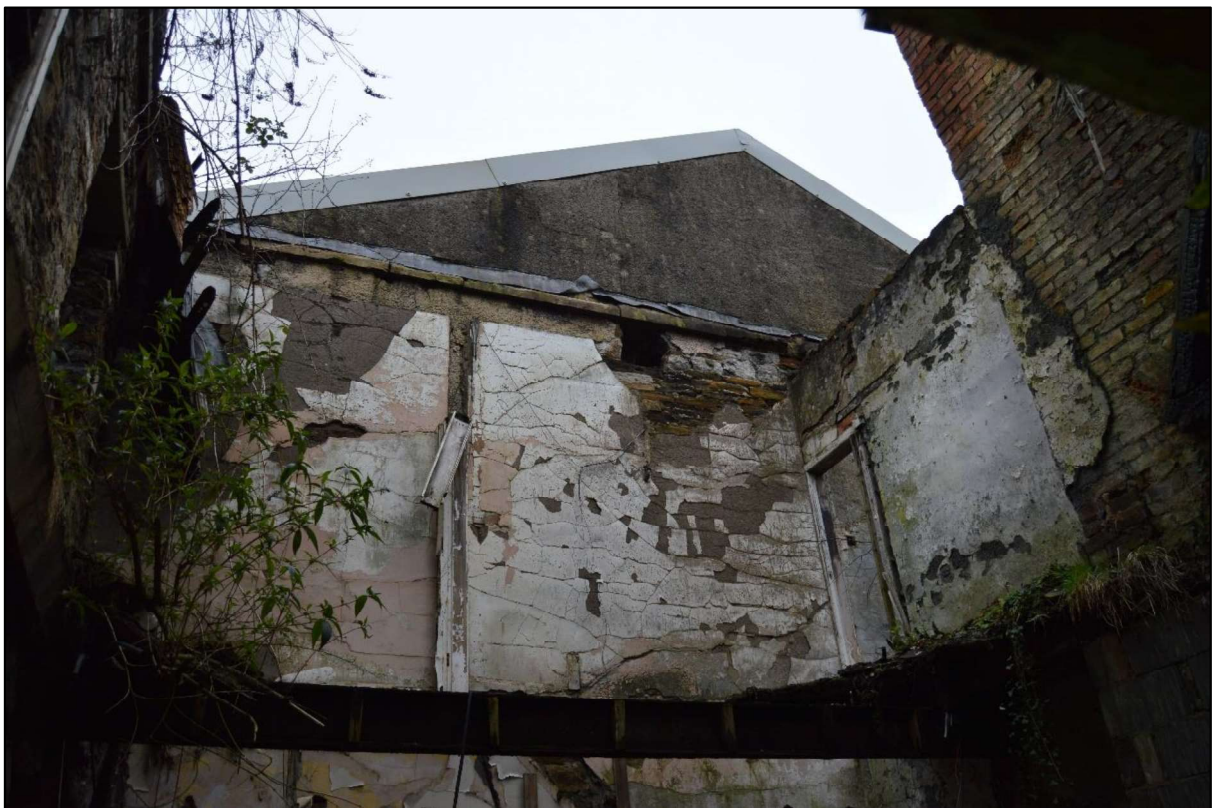
Photo 90: View north east towards the south west gable of the north range from ground floor level within the north unit of the former cottage.
