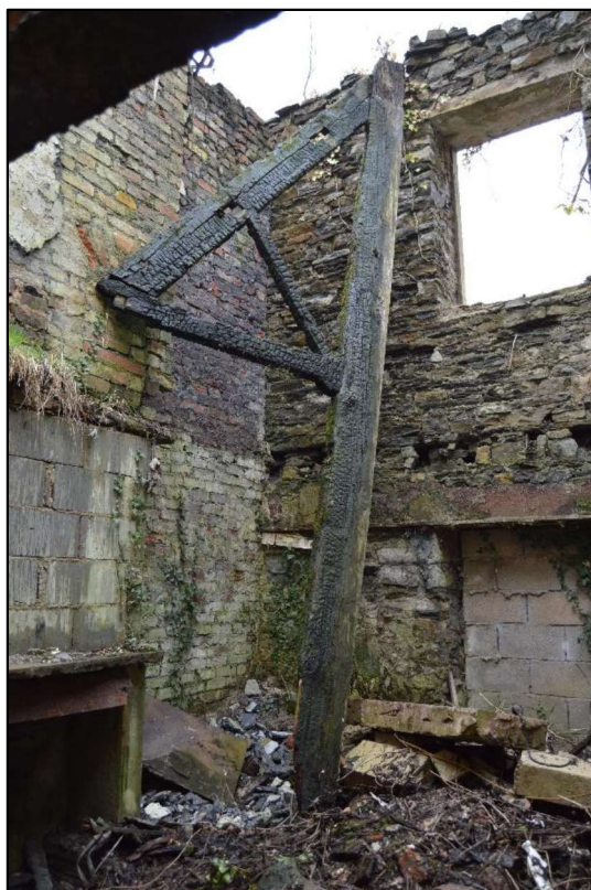
Photo 87: View of charred remains of a timber king post roof truss within the north unit of the former cottage.
