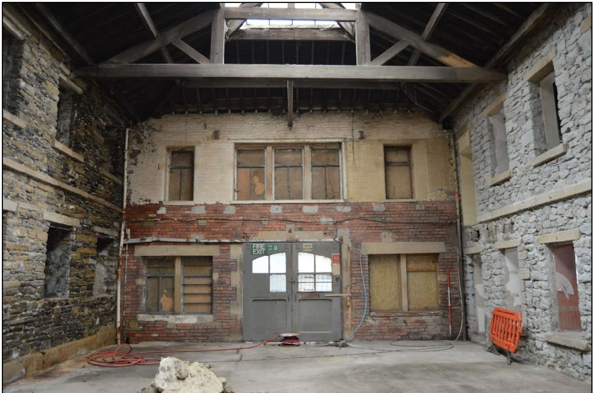
Photo 63: View north east along the central range.
