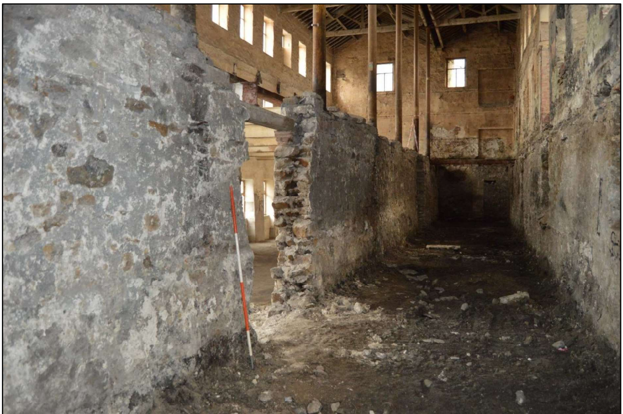
Photo 46: View south along the north section of the south range at lower ground floor level.
