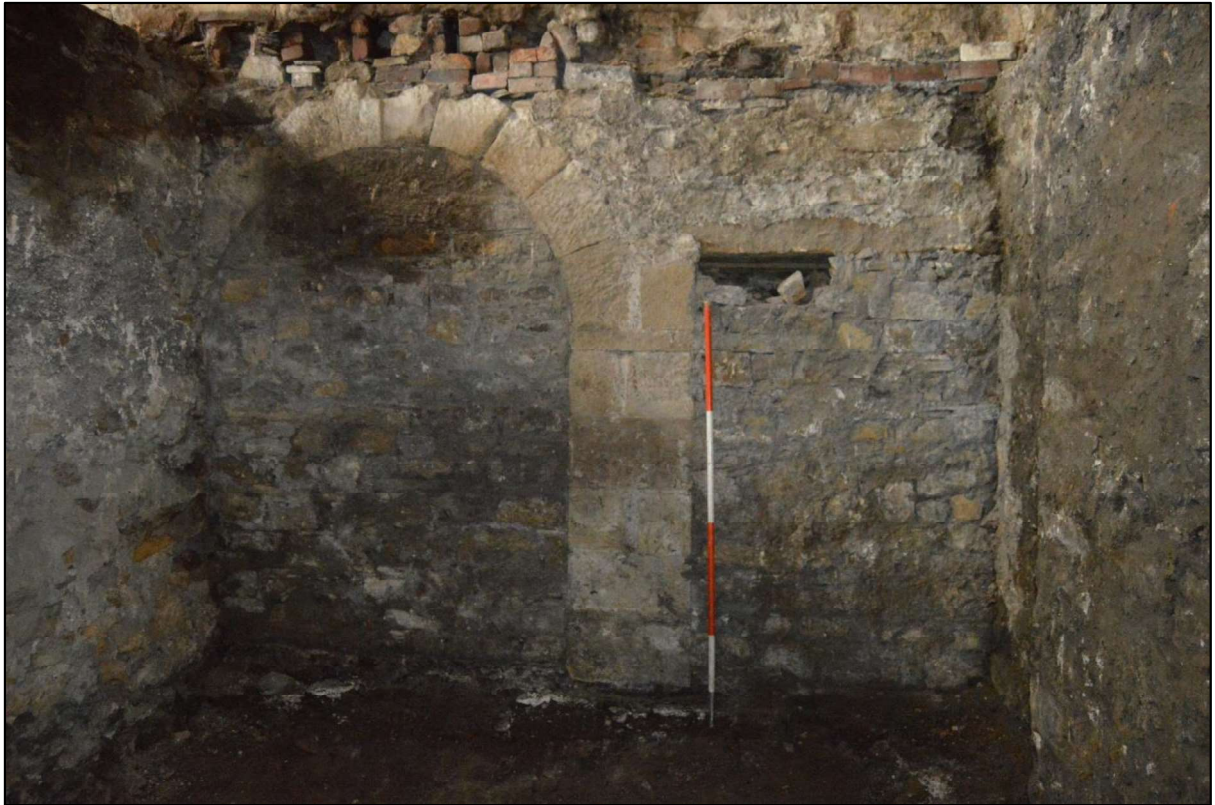
Photo 43: View of blocked door and arched opening to the south west gable.
