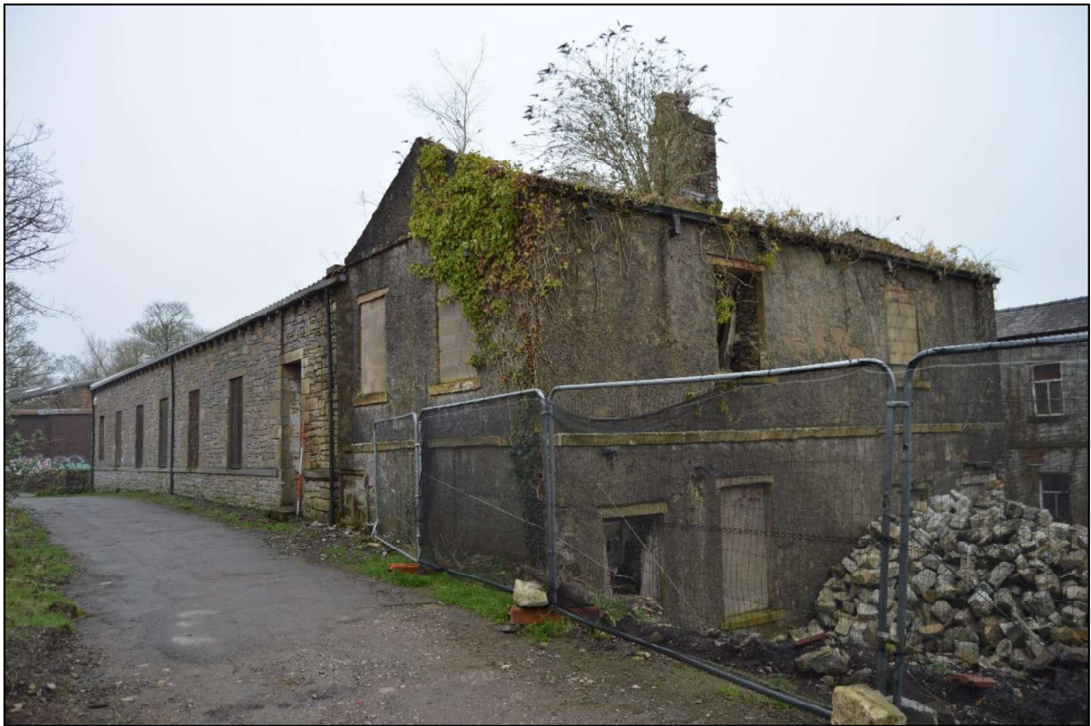
Photo 11: View of the north range and former cottage from the east.
