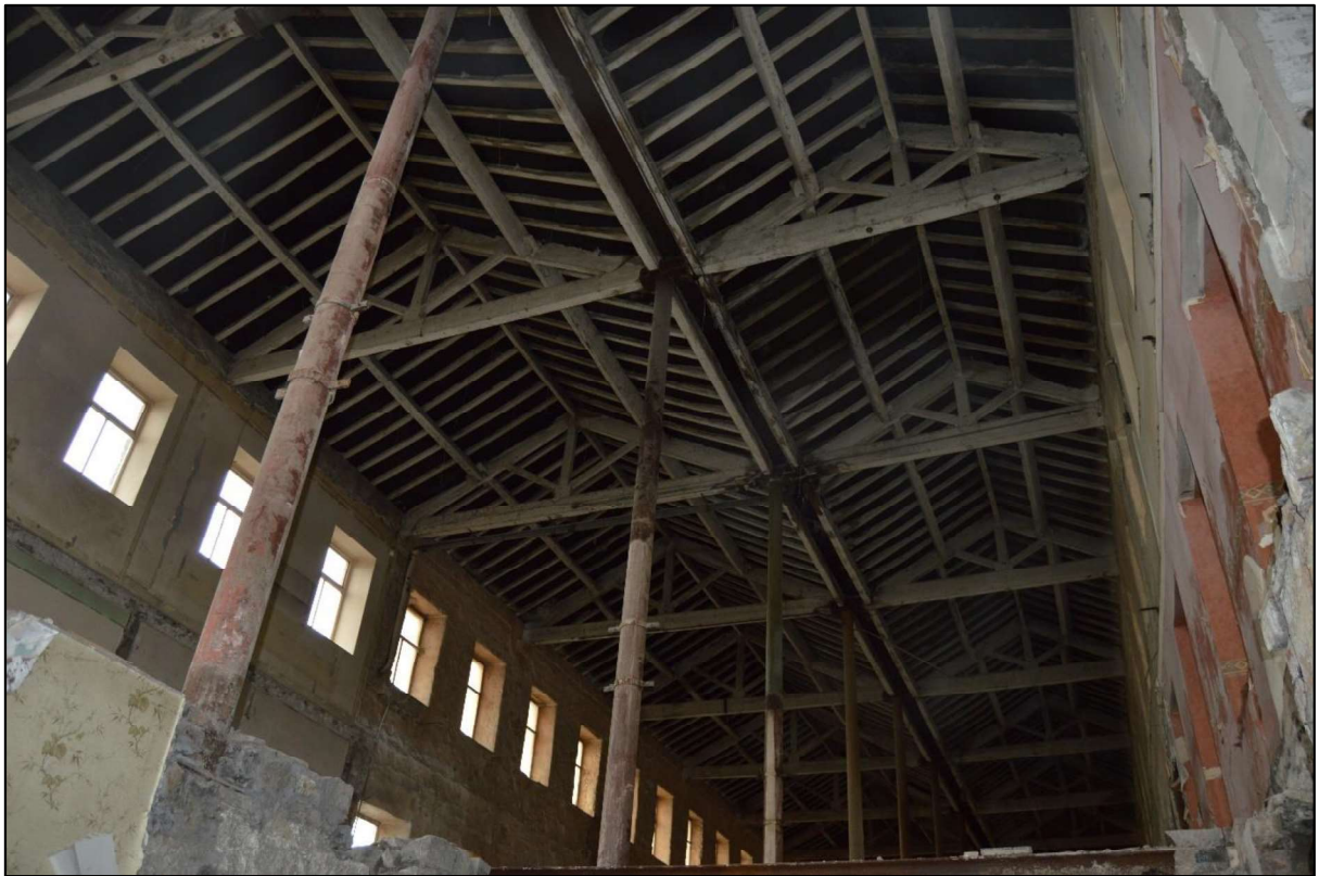
Photo 57: View of the roof structure over the south range.
