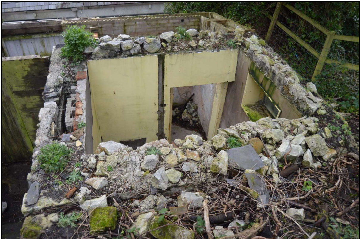
Photo 21: View of the smaller outbuilding to the south west of the south range from the north.
