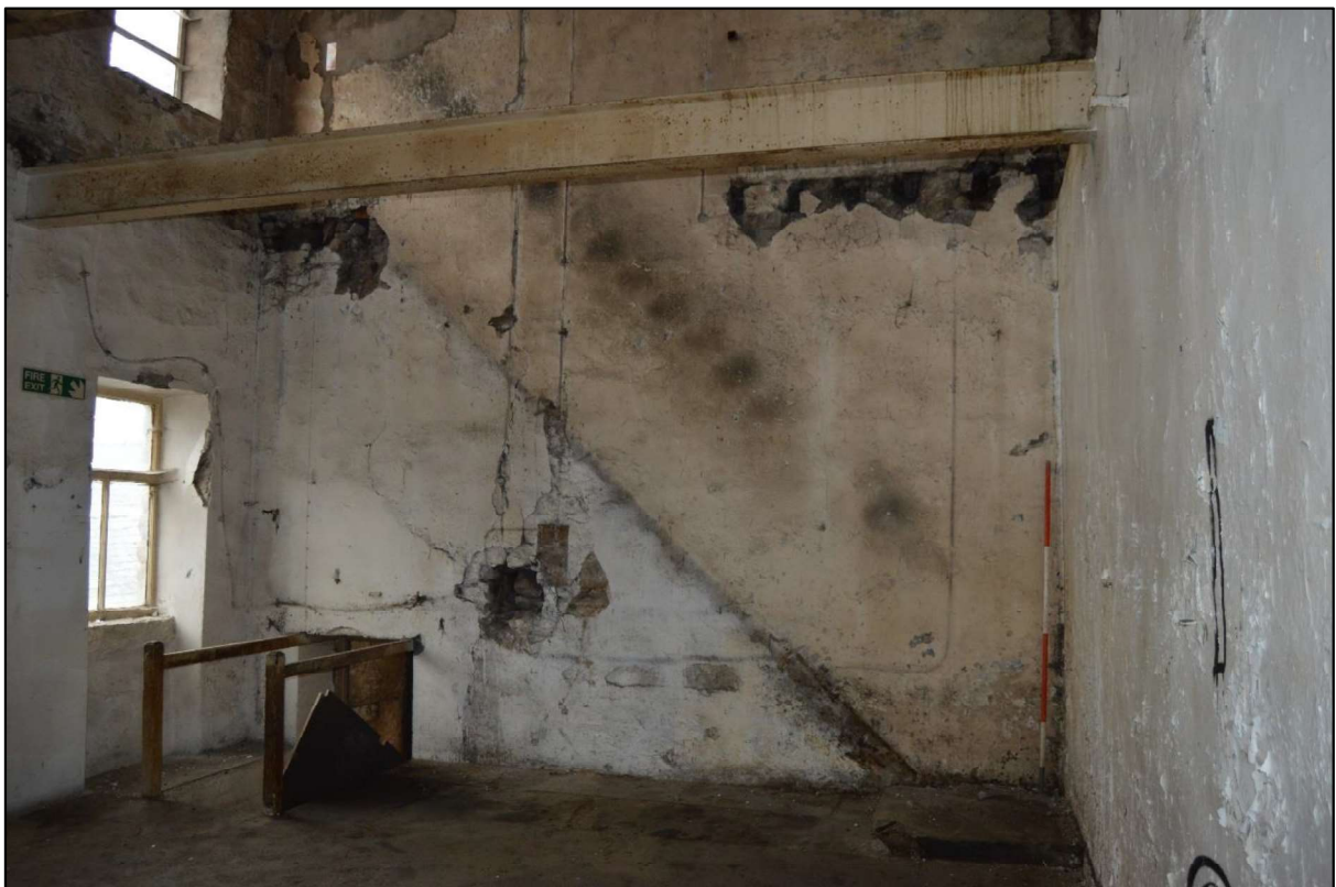
Photo 28: View of the former stair position to the south west gable at lower ground floor level to the south range.
