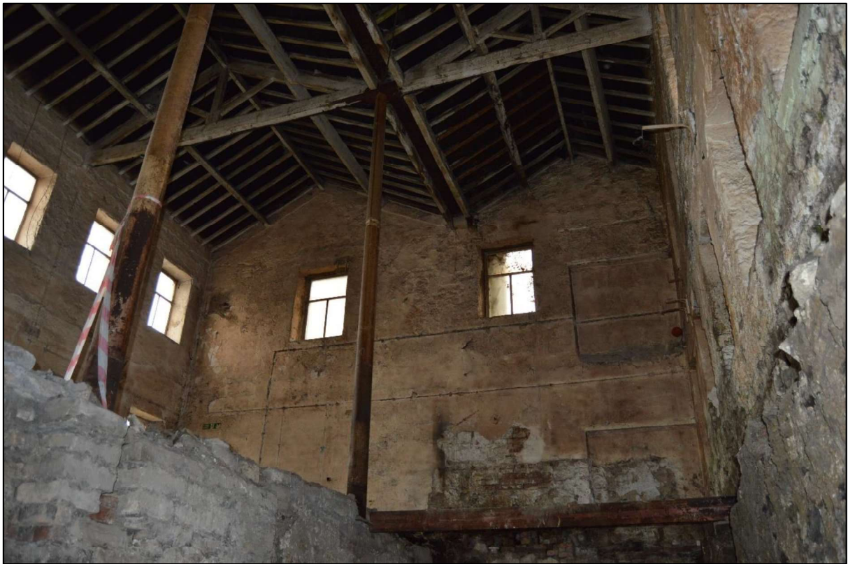
Photo 45: View south west towards the upper levels of the south west gable ends.
