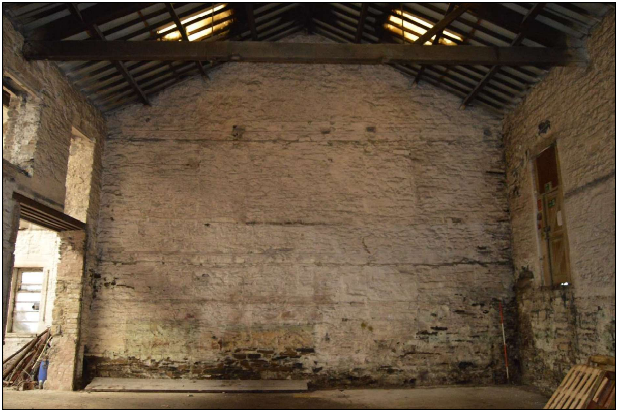
Photo 69: View of the south west gable end of the north range.
