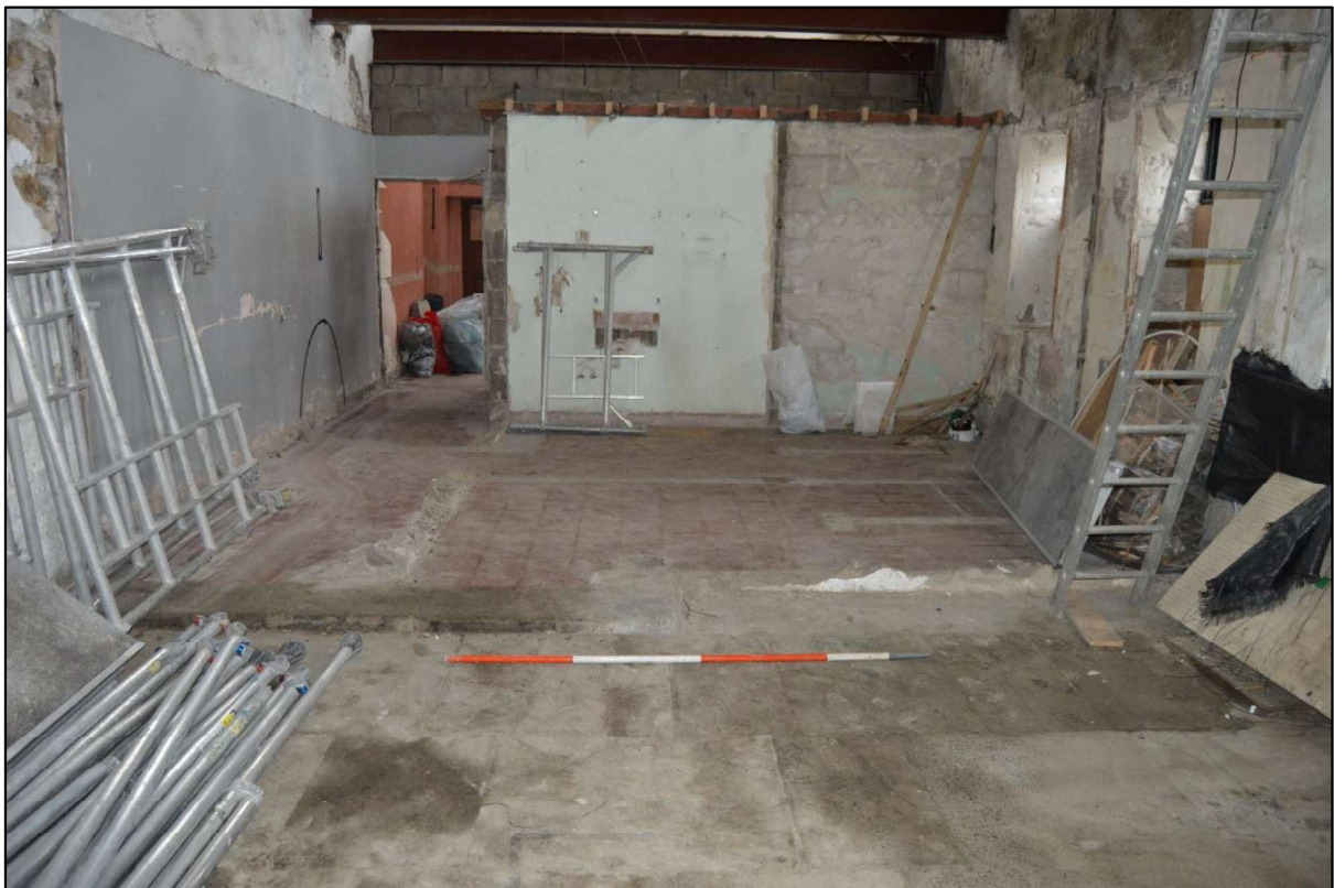
Photo 32: View of former partition locations to the north east end of the south range at lower ground floor level.
