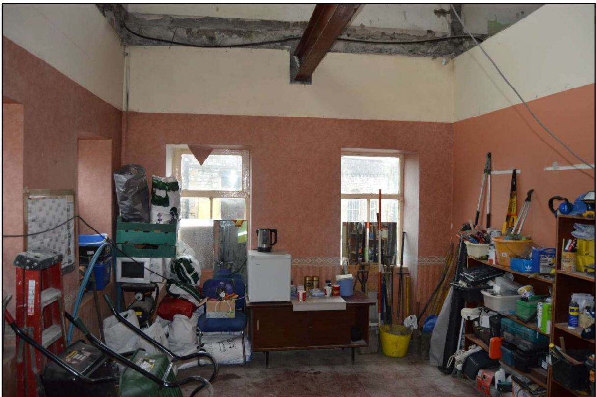
Photo 40: View south east within the north east unit at lower ground floor level to the south range.
