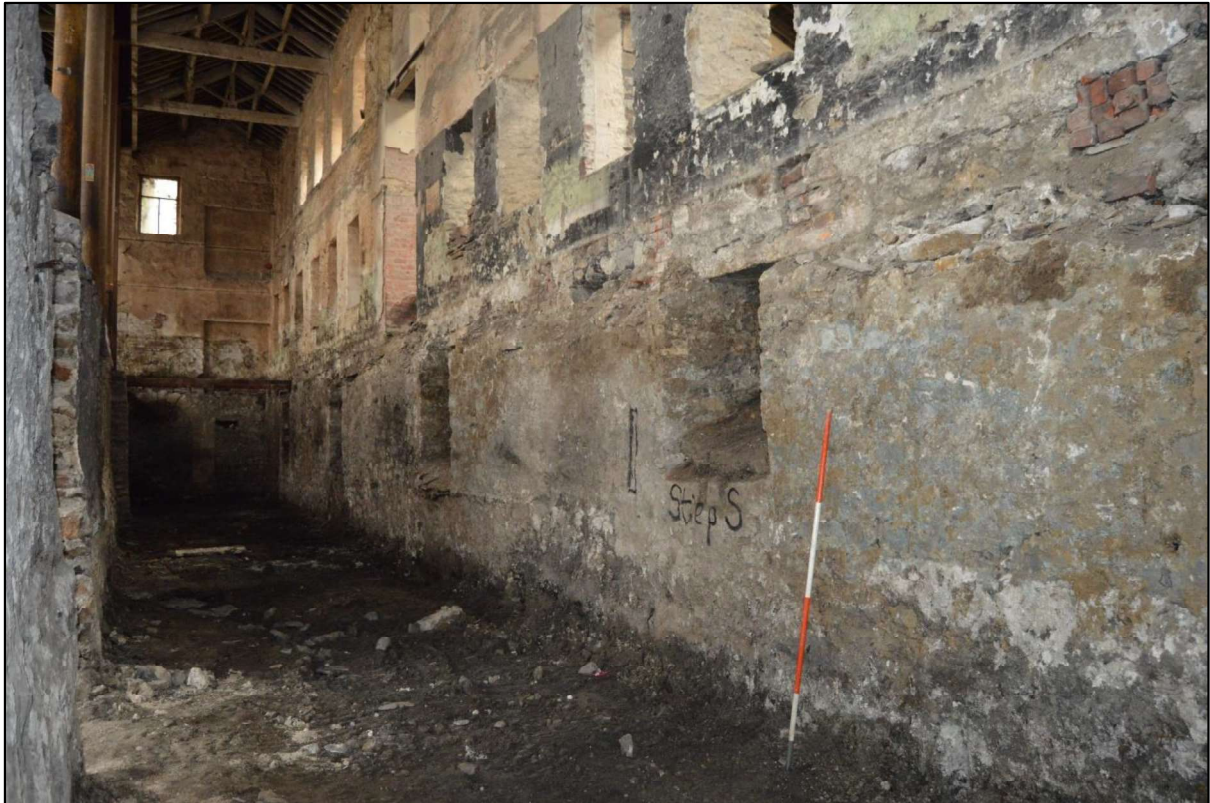
Photo 47: View west along the north section of the south range at lower ground floor level.
