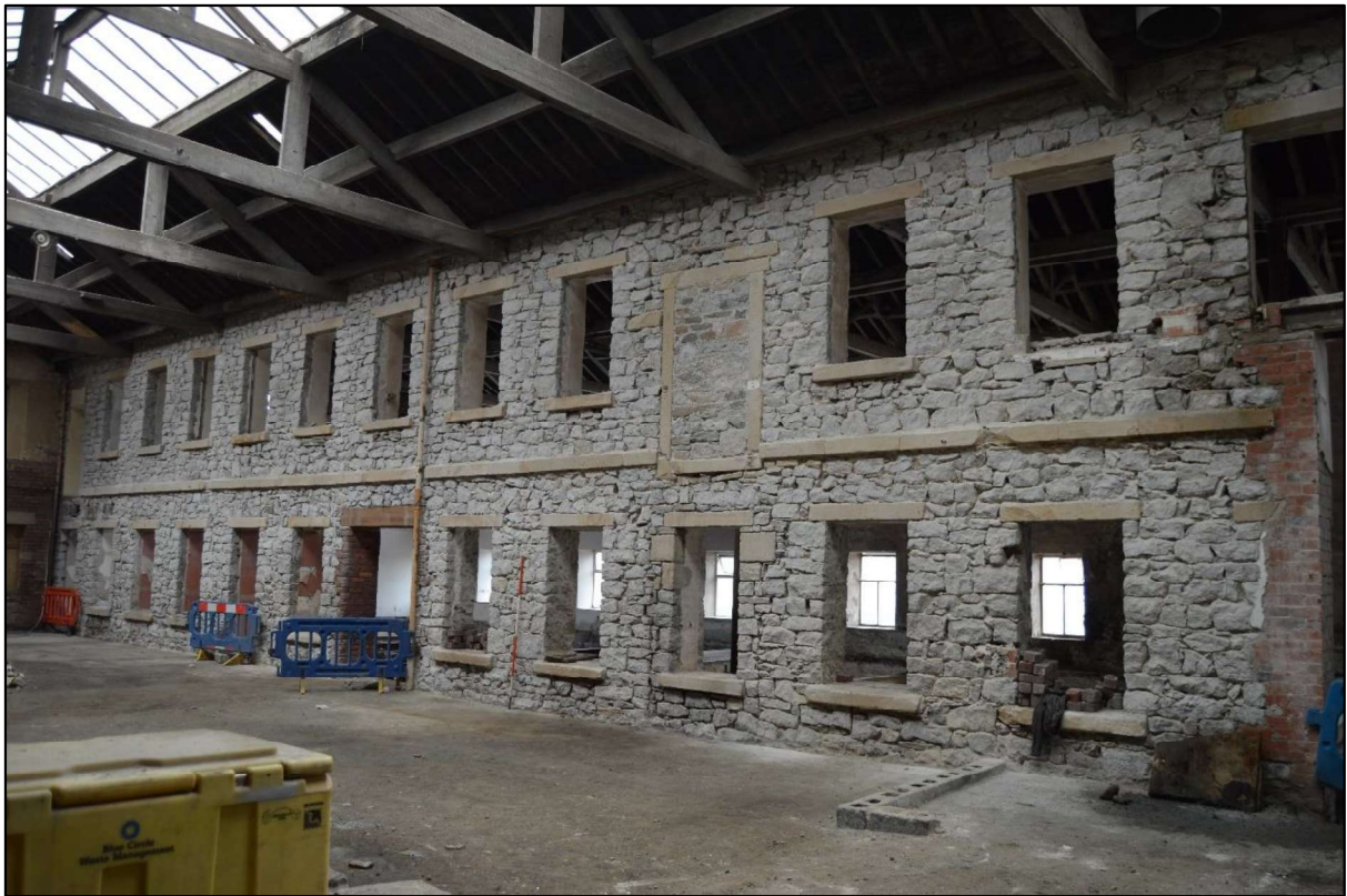
Photo 61: View east along the central range.
