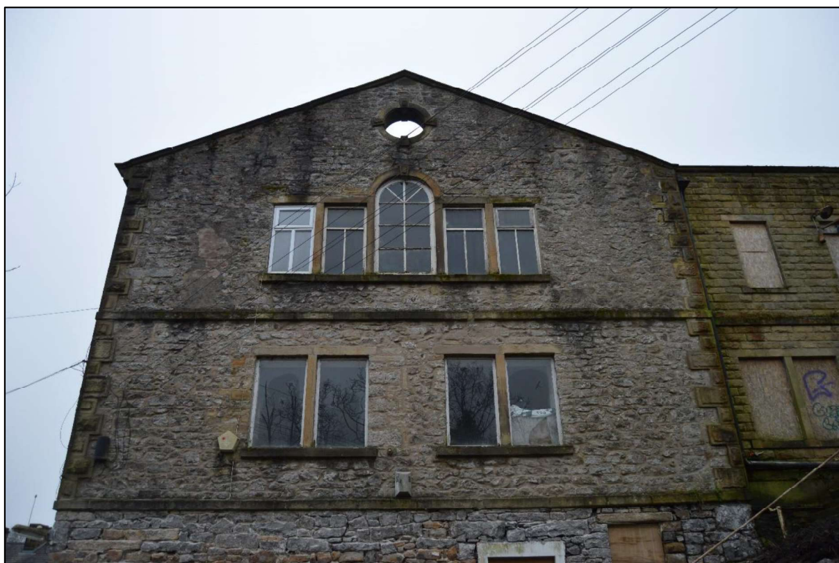
Photo 02: View of the upper windows to the north east gable end of the south range.
