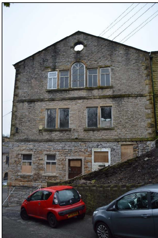
Photo 01: View of the North east gable end of the south range.
