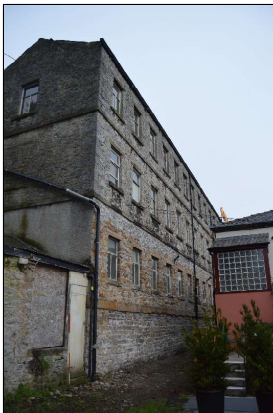
Photo 25: View of the south east elevation of the south range from the south west.
