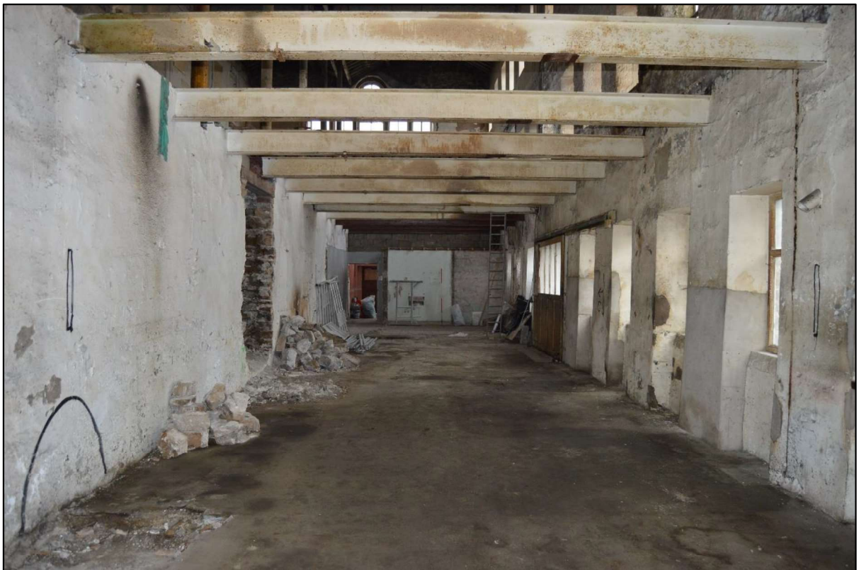
Photo 30: View north east along the lower ground floor of the south range.
