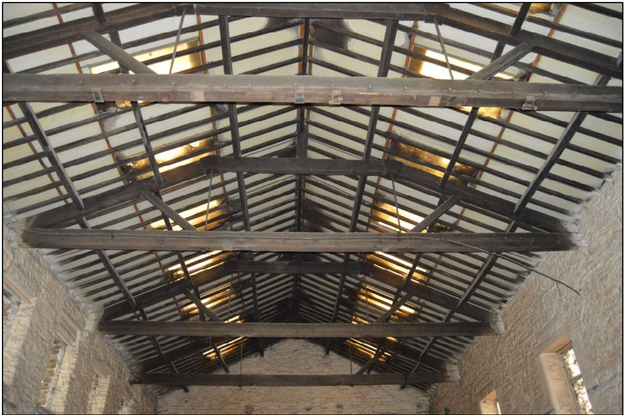
Photo 77: View of roof structure over the north range.
