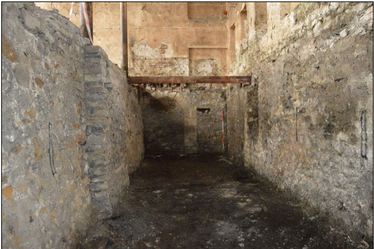
Photo 42: View south west at lower ground floor level within the northern section of the south range.
