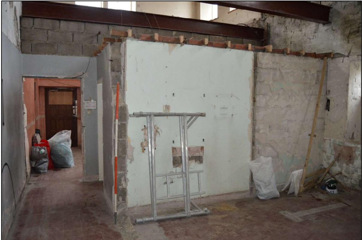
Photo 35: View of modern partitions to the north east end of the south range at ground floor level.
