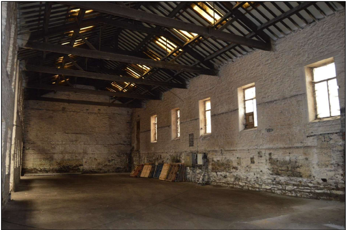
Photo 71: View west along the north range.
