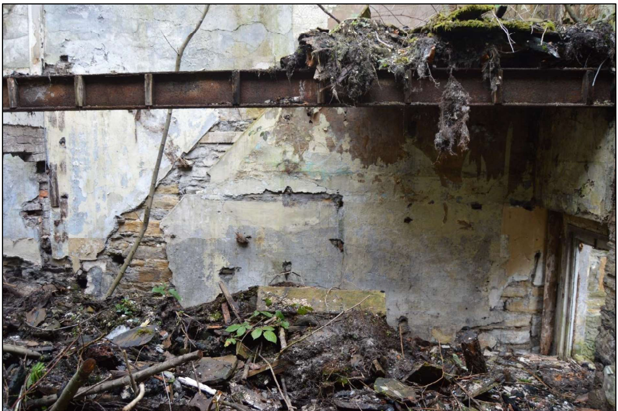
Photo 80: View north east at ground floor level within the south unit of the former cottage.
