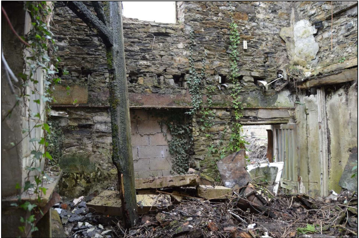
Photo 83: View south west at ground floor level within the north unit of the former cottage.
