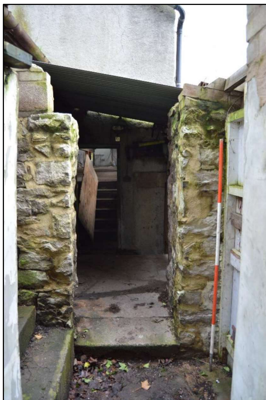
Photo 95: View north east along the passage between the outbuildings to the south west of the south range.
