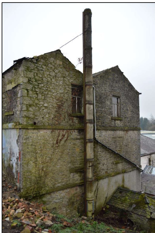
Photo 17: View of the south west elevation of the south range.
