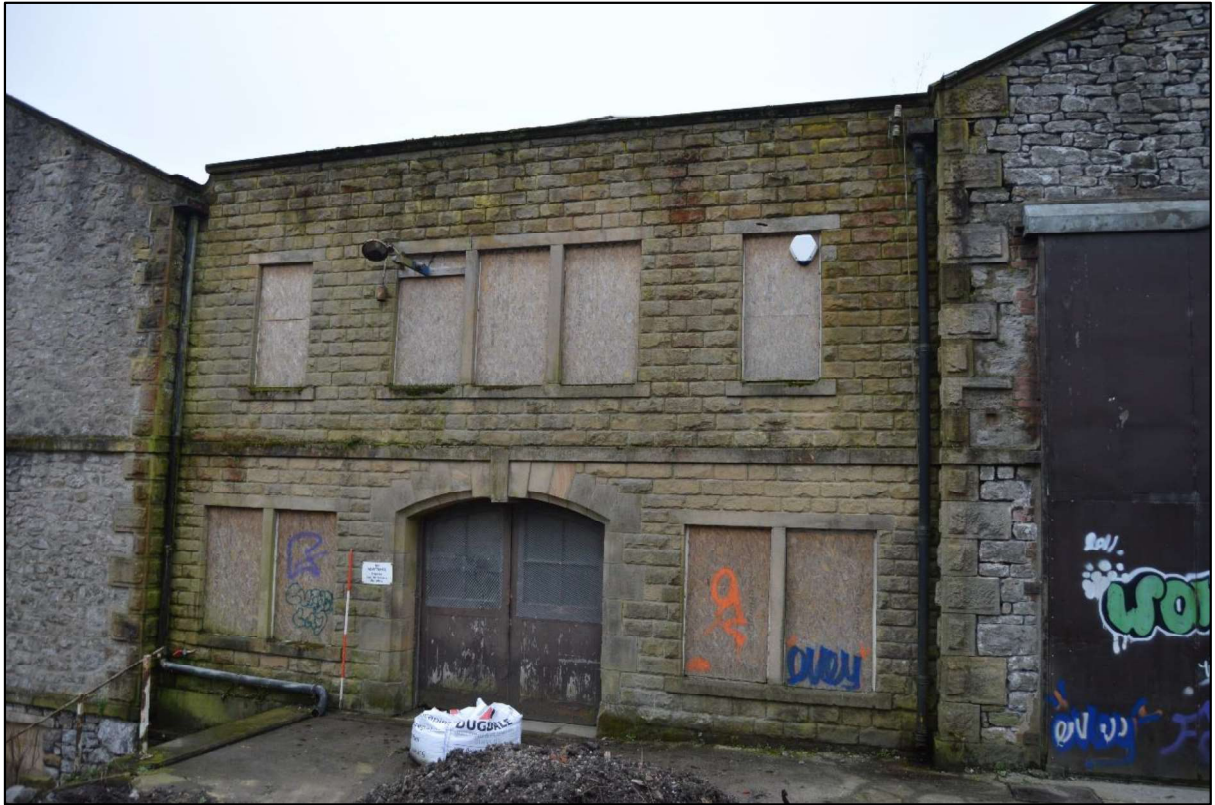
Photo 05: View of the north east elevation of the central range.
