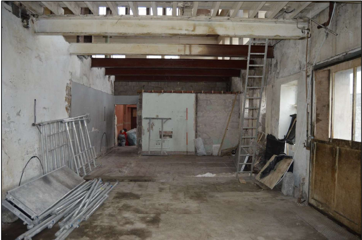
Photo 31: View north east towards to north east gable at lower ground floor level within the north range.
