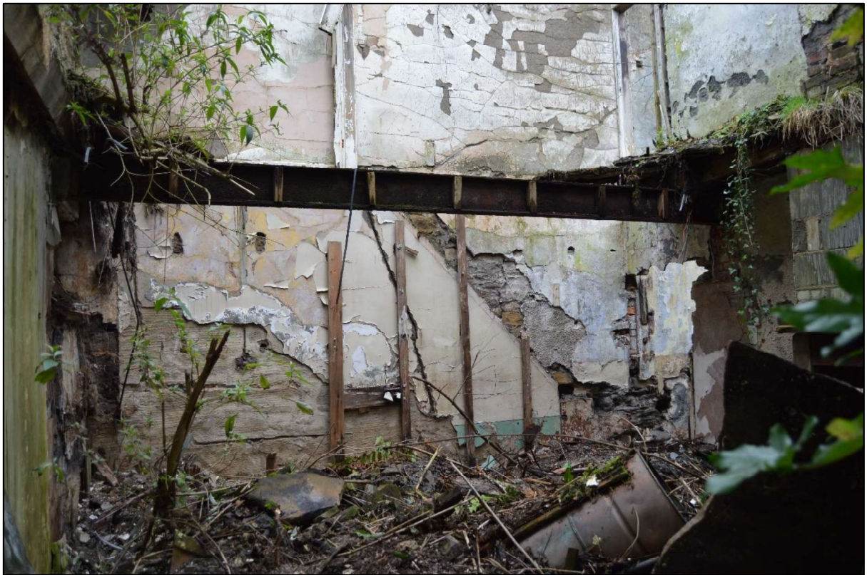
Photo 89: View north east at ground floor level within the north unit of the former cottage.
