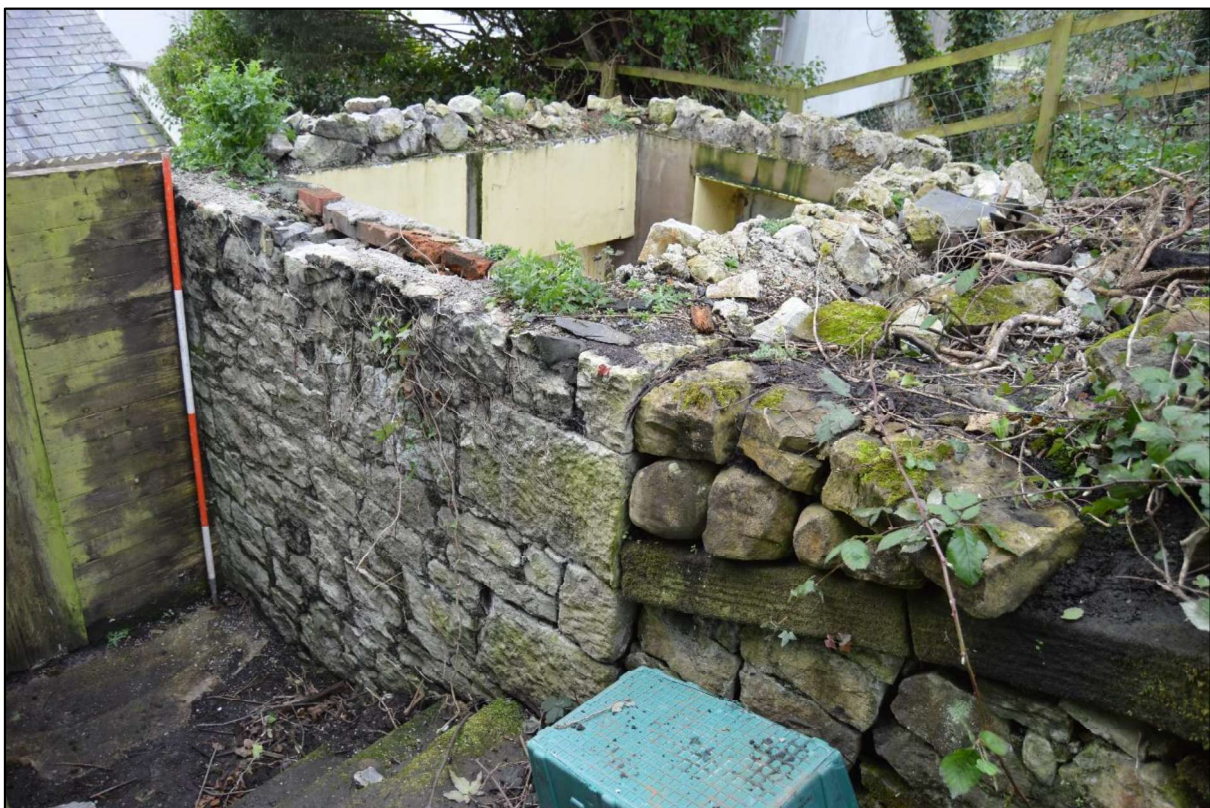
Photo 22: View of the smaller outbuilding to the south west of the south range from the north.
