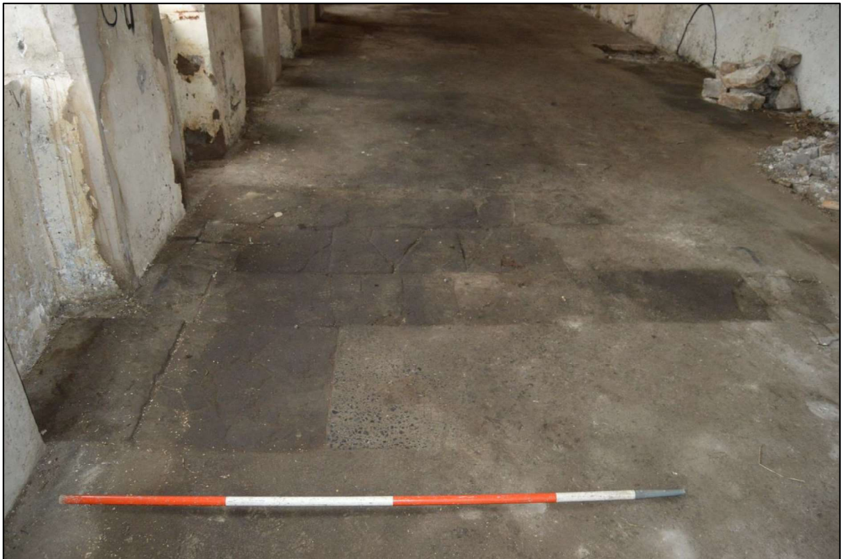
Photo 33: View of stone flag flooring at lower ground floor level to the south range.
