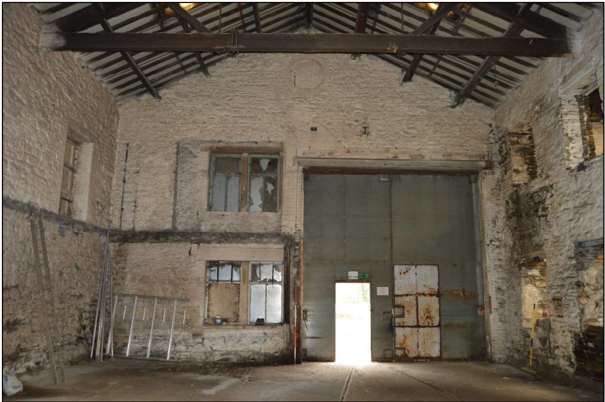
Photo 73: View of the north east gable of the north range.
