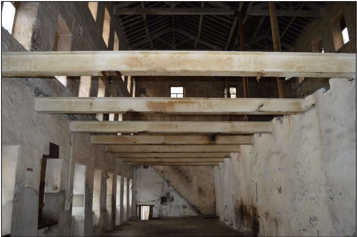
Photo 29: View of the remnants of the ground floor structure above the lower ground floor of the south range.
