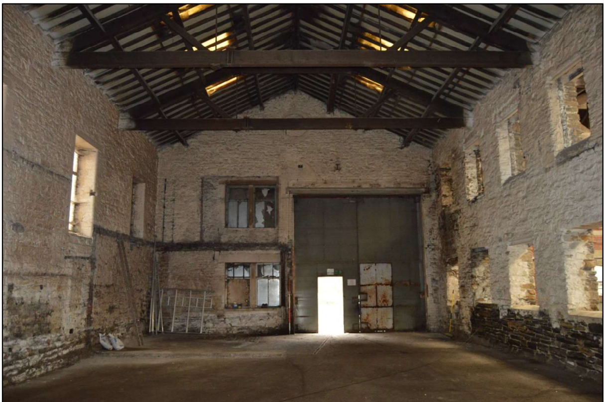
Photo 72: View north east along the north range.
