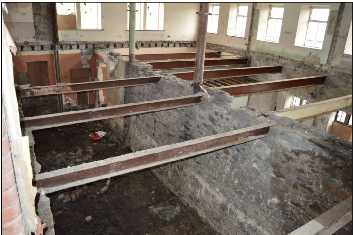
Photo 56: View east along the south range from ground floor level.
