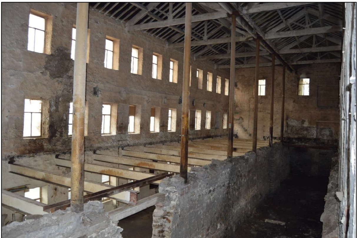
Photo 54: View south west along the south range from ground floor level.
