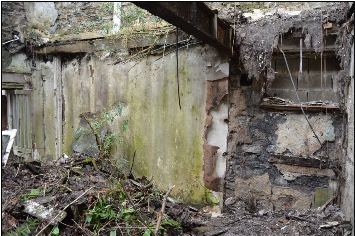
Photo 85: View west at ground floor level within the north unit of the cottage.
