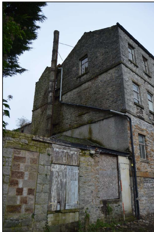
Photo 24: View of the south west elevation of the south range from the south.
