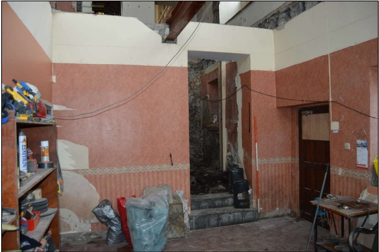
Photo 41: View north within the north east unit at lower ground floor level to the south range.
