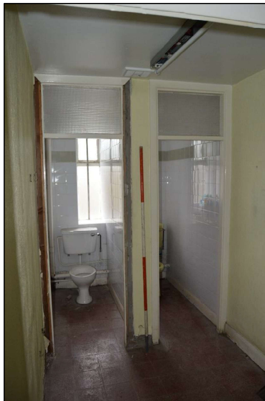
Photo 36: View south east within the WC's at lower ground floor level within the south range.
