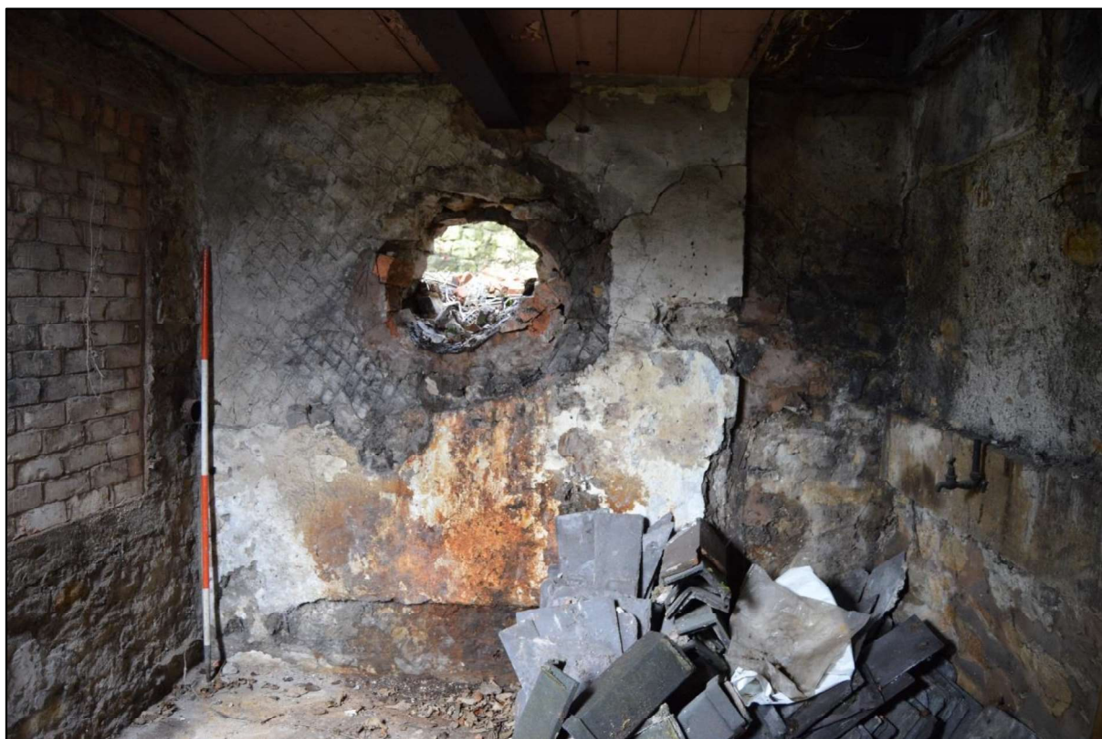
Photo 96: View north west within the adjoining outbuilding to the south west of the south range.
