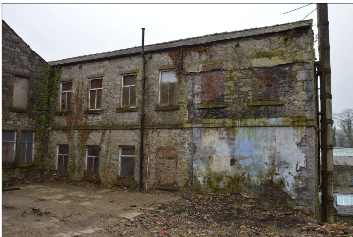
Photo 16: View of the north west elevation of the south range.
