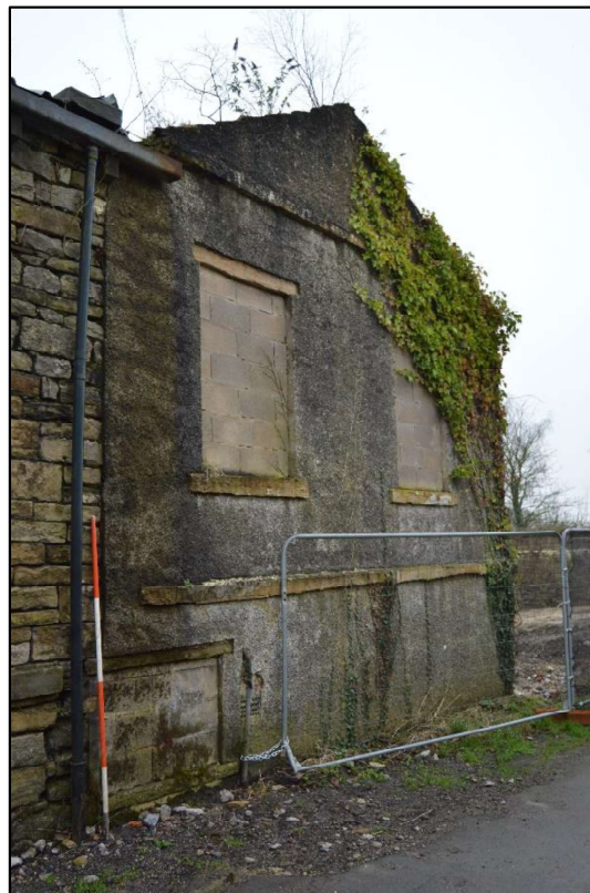
Photo 12: View of the north west gable end of the former cottages.
