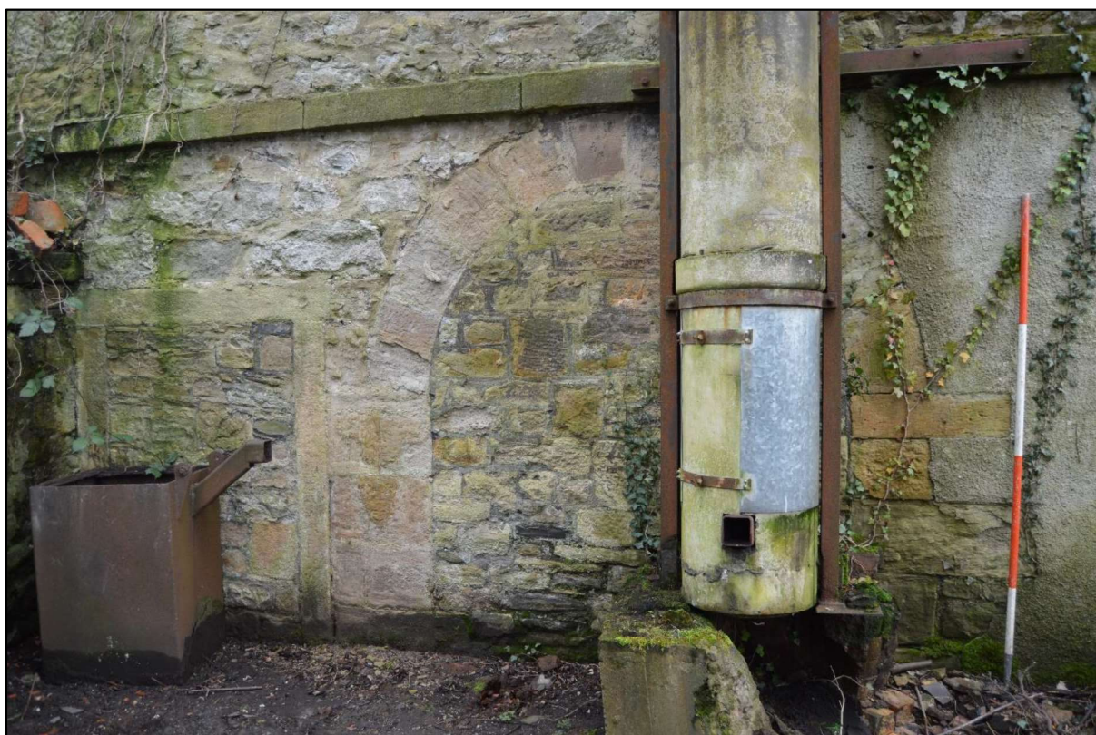
Photo 18: View of blocked up openings at lower ground floor level to the south west elevation of the south range.
