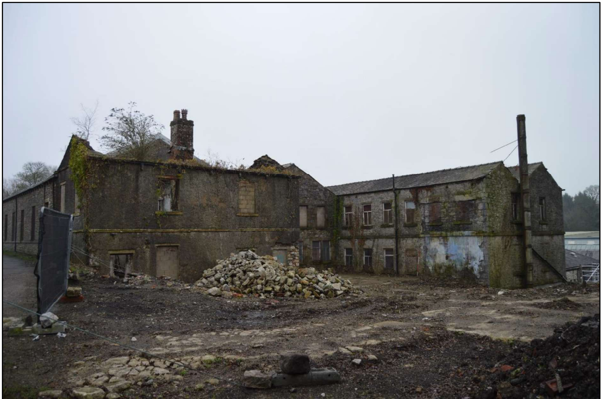
Photo 13: View of the former print works from the east.
