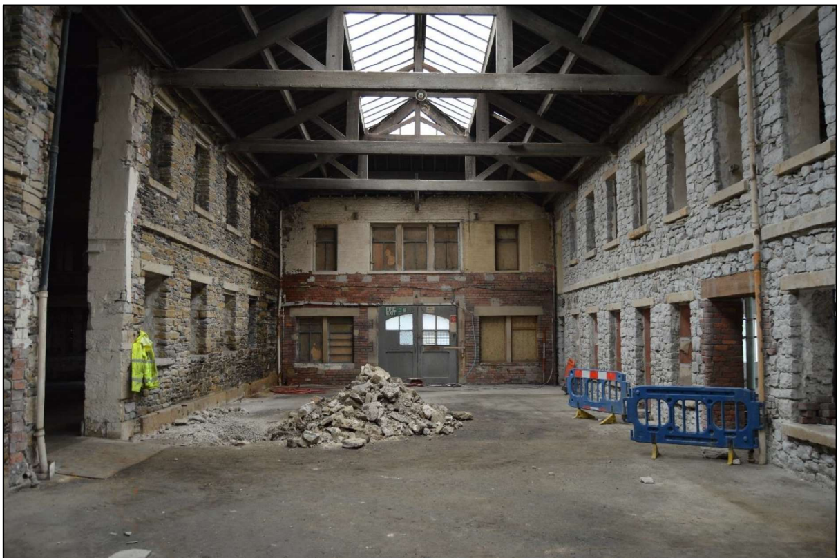
Photo 62: View east along the central range.
