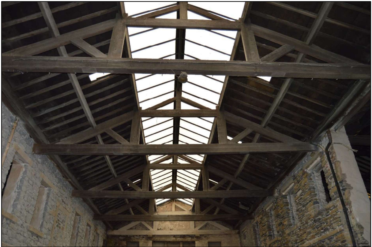
Photo 67: View of roof structure over the central range.
