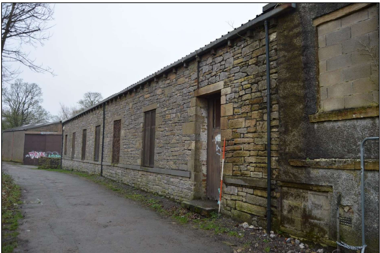
Photo 10: View of the north west elevation of the north range from the east.
