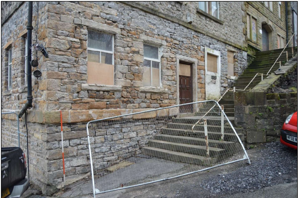
Photo 04: View of the lower ground floor entrance and steps to the north east gable end of the south range.
