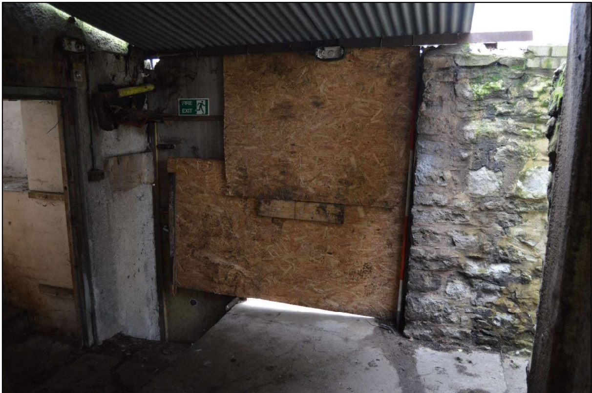
Photo 97: View south east within the adjoining outbuilding to the south west of the south range.
