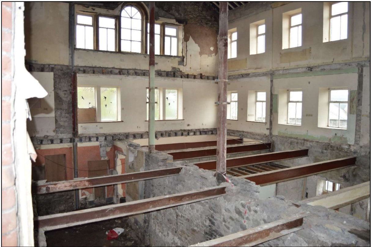
Photo 55: View east along the south range from ground floor level.
