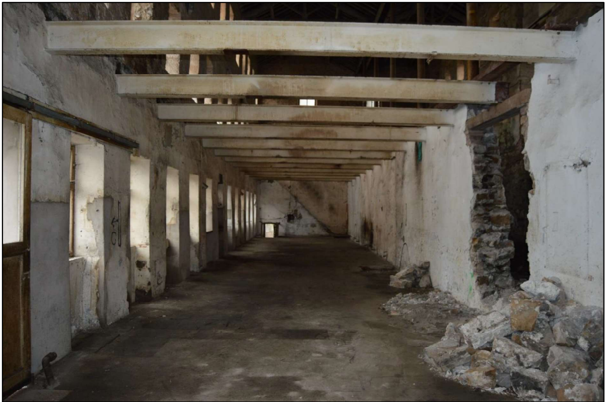
Photo 27: View south west along the lower ground floor of the south range.
