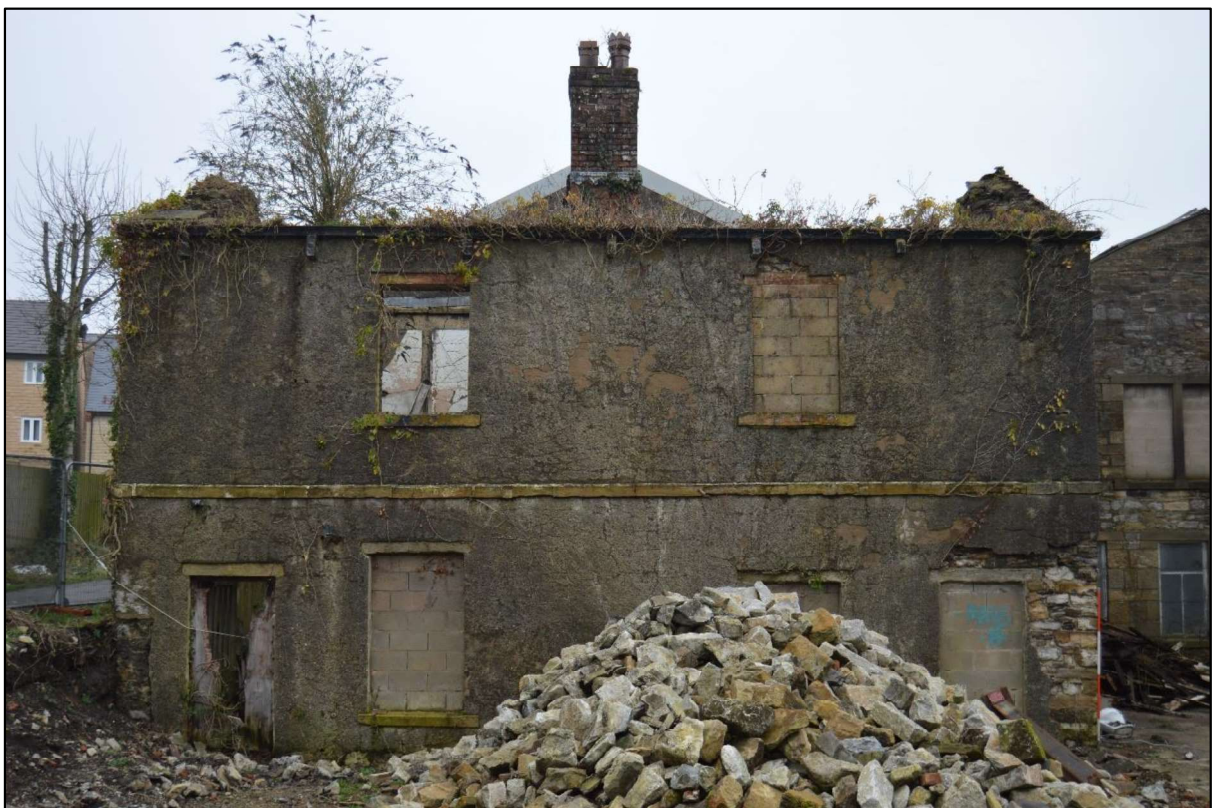
Photo 14: View of the south west elevation of the former cottages.
