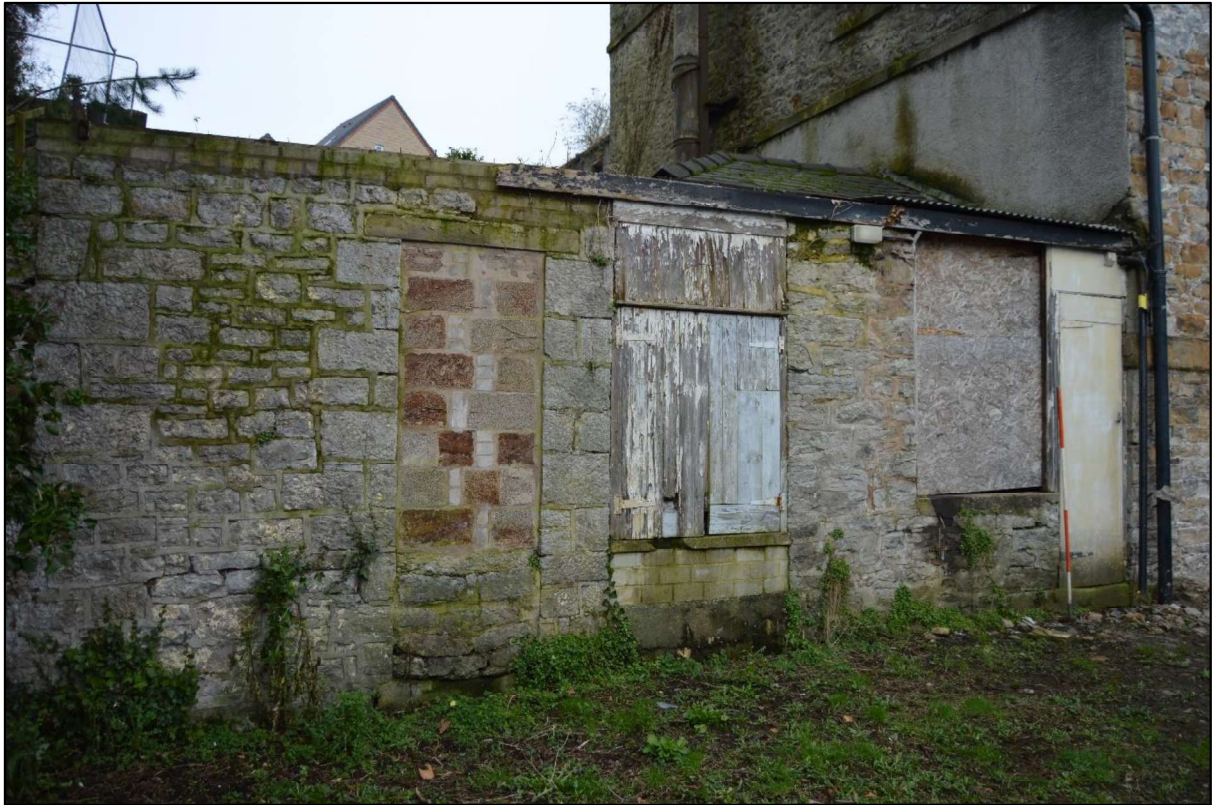
Photo 23: View of the outbuildings to the south west of the south range from the south.
