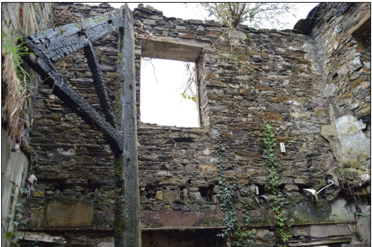
Photo 84: View south west towards first floor level from ground floor level within the north unit of the former cottage.
