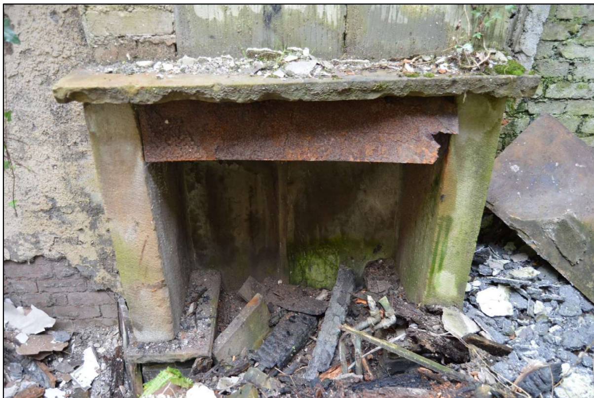
Photo 88: View of the fireplace at ground floor level withing the north unit of the former cottage.
