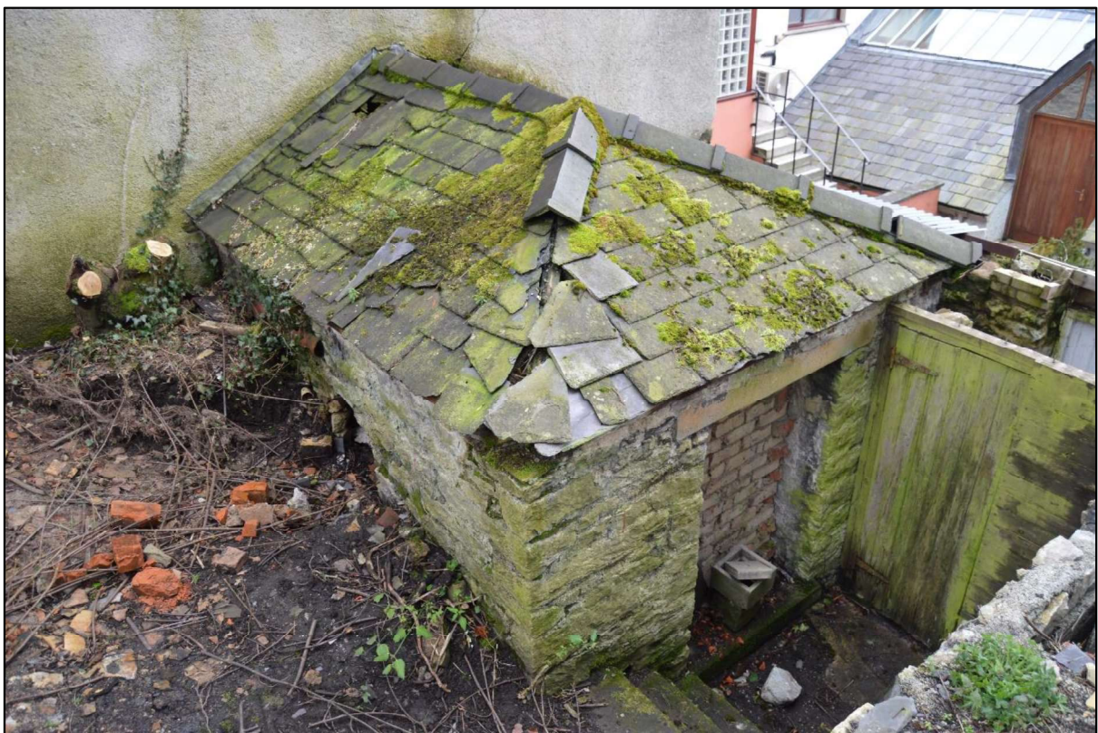
Photo 20: View of the adjoining out building to the south east of the south range from the north.
