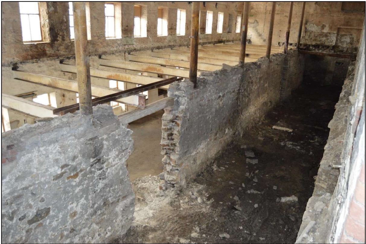
Photo 53: View south west along the south range from ground floor level.
