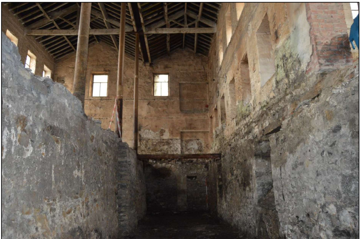
Photo 44: View south west along the north section of the south range.
