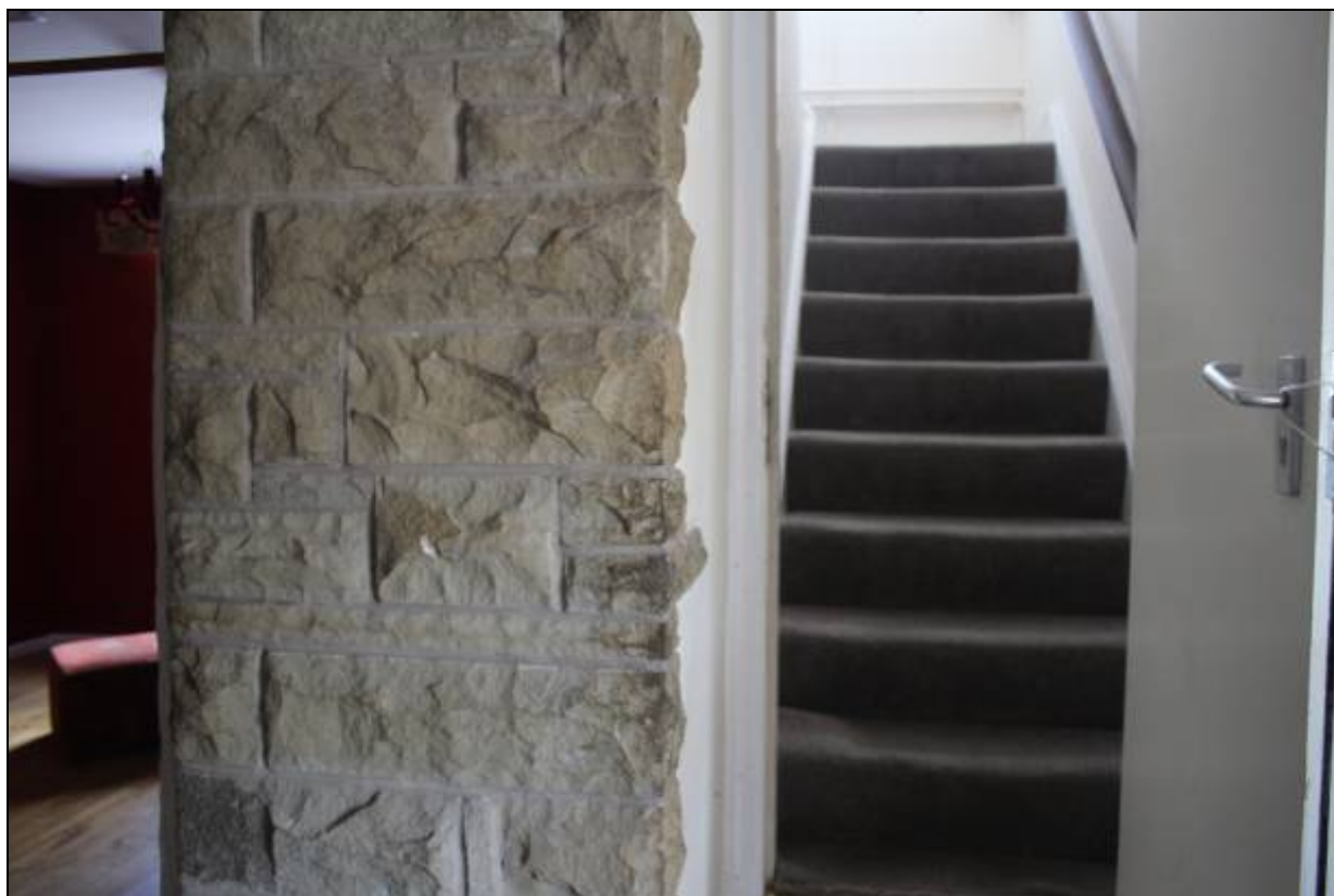
10. Present staircase dates from between 1905 and 1926
