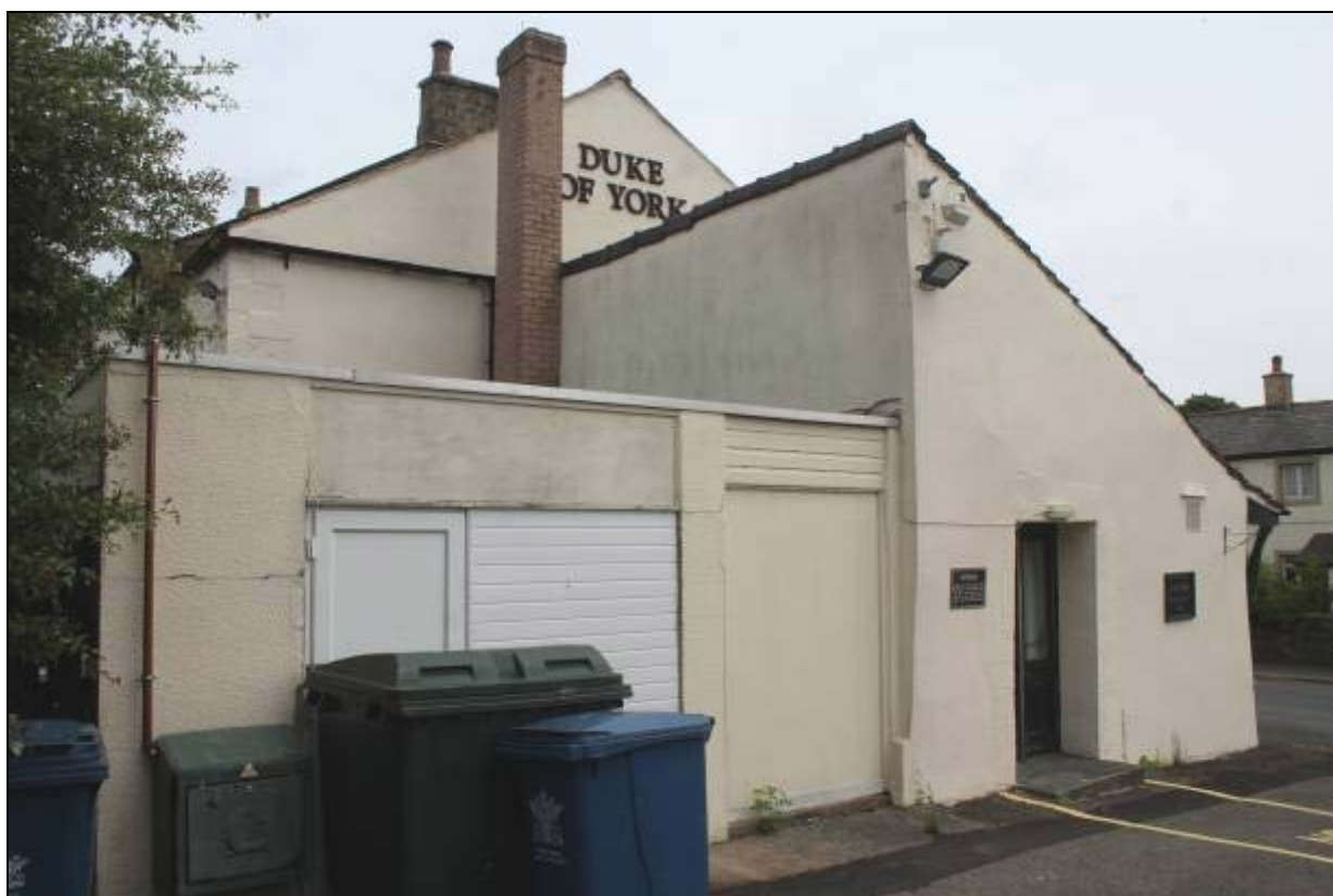
9. Flat-roofed building behind the dining room extension with its single-pitch roof
