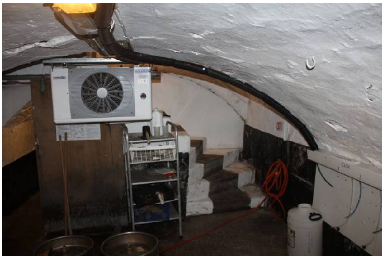
13. The central vaulted cellar room, with stone steps
