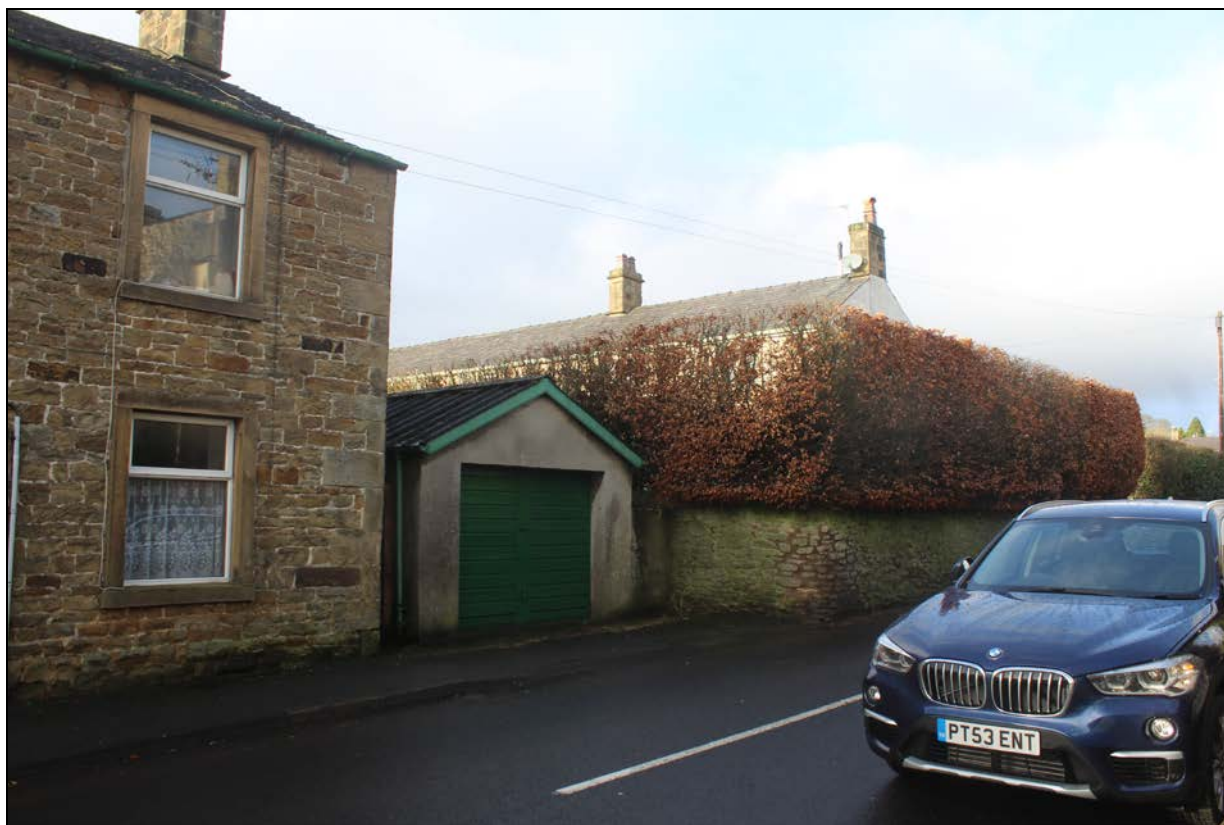
16. Townley House as viewed from Main Street, opposite the Duke of York
