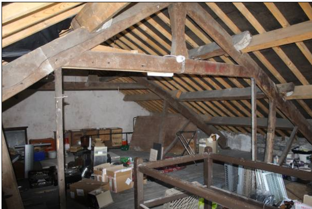
12. The attic is a single-space spanned by a pair of wide kingpost trusses
