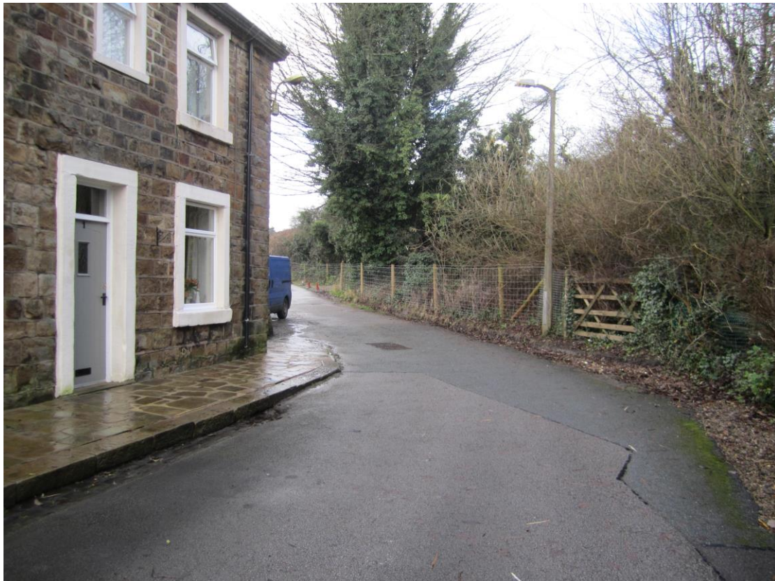
2 Bank Cottages looking west
