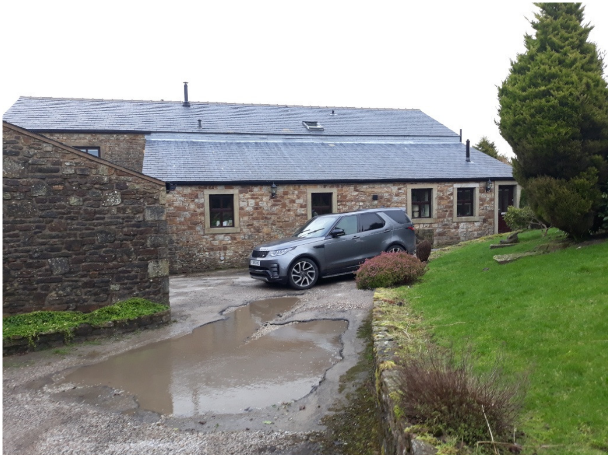
West Elevation showing lean – to where rooflights to be inserted.
