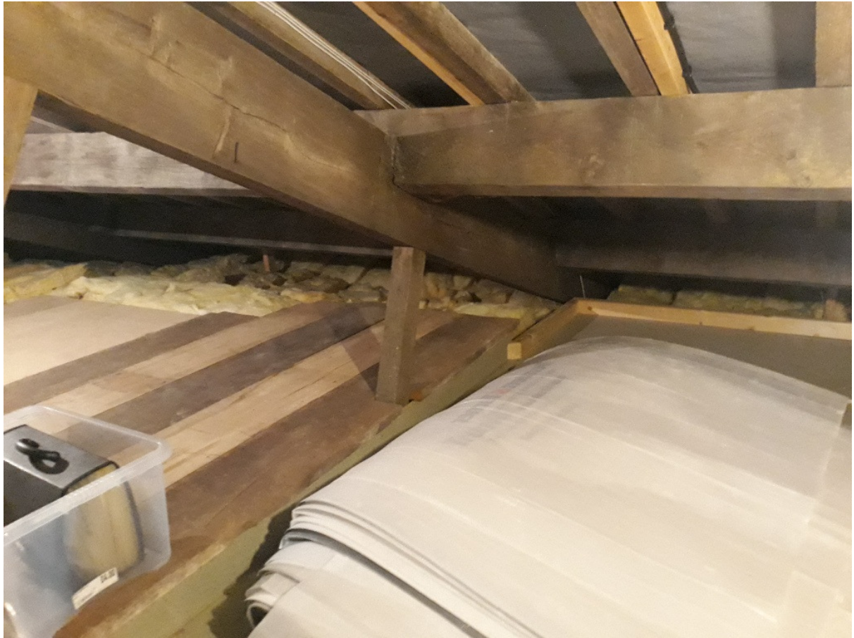
Internal roof space with new timbers and roofing felt visible.
