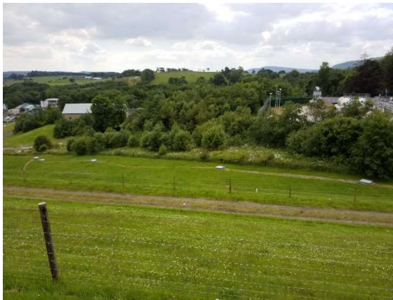
Figure 3: View from reservoir embankment looking west, G3 (foreground) and G1 (centre)
