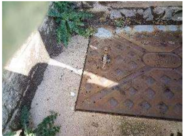
Bat droppings in the corner of Building 2 and 3
