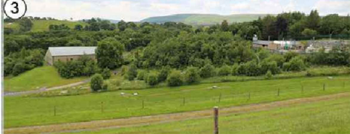
View looking at northern side of the Rapid Gravity Filter Site
