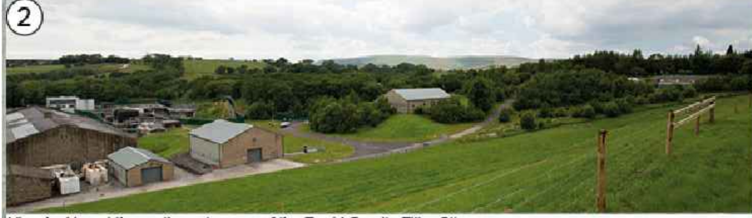
View looking at the north-east corner of the Rapid Gravity Filter Site. Image illustrates the expansive built form set out across the water treatment works site.
