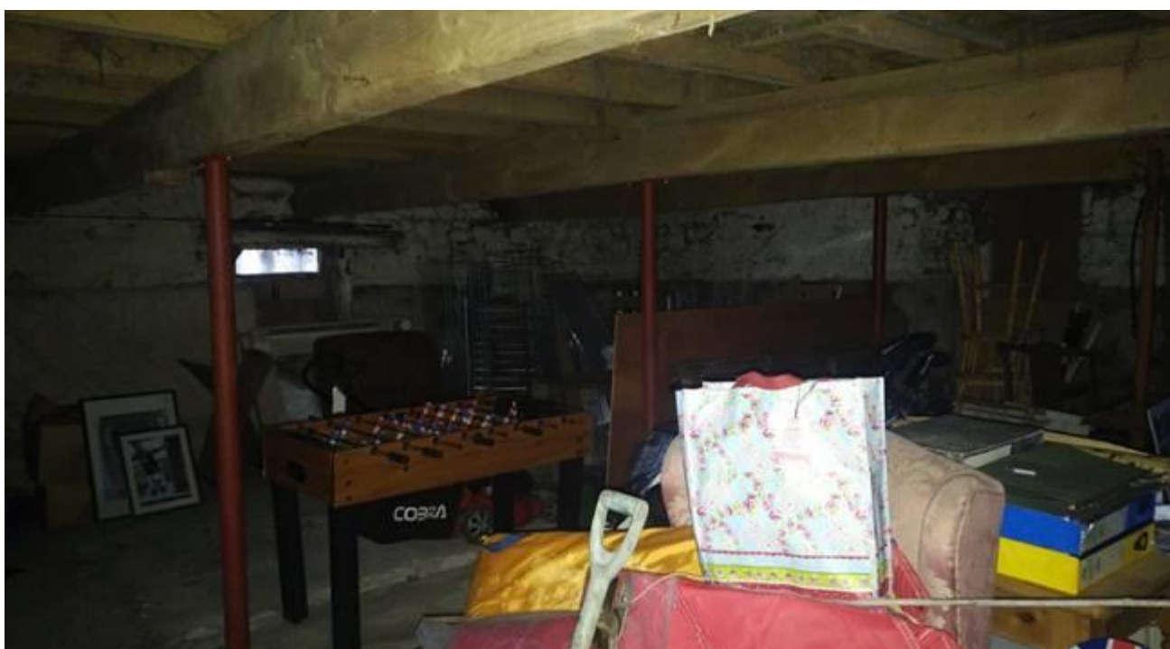
Figure 9) Inserted loft floor over shippon in main barn with steel posts
