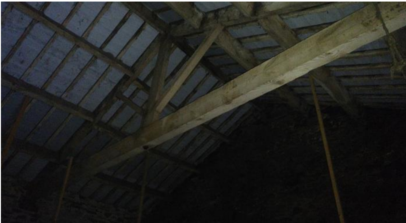
Figure 10) Kingpost roof truss with butted purlins in main barn
