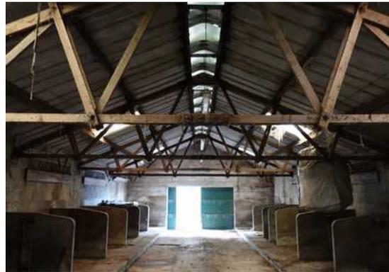
A detached single storey concrete block shippon with double pitched corrugated fibreboard roof is present to the north of the barn. The building has no obvious gaps or crevices suitable for roosting bats. Fascia boarding where present is close fitting. Roof lights are present and allow considerable light penetration.
