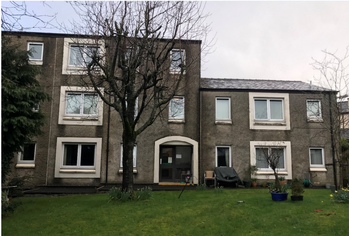
View of the door offering access to the proposed store
