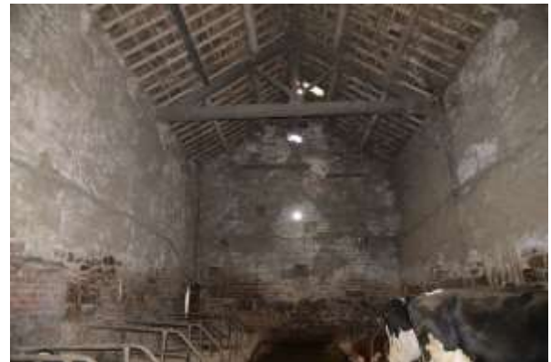
Plate 26 Interior of the barn, looking north
