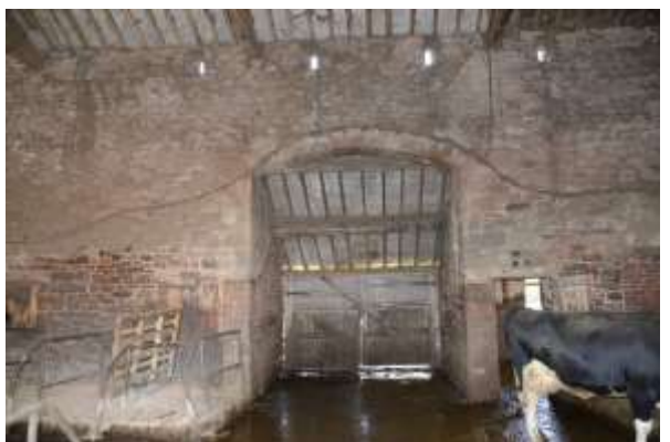
Plate 28 Interior of the threshing door opening through the southwest wall
