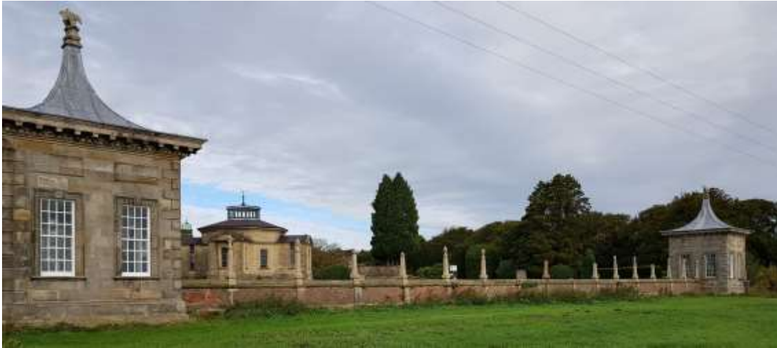
Plate 6 Garden wall and pavilions, looking north
