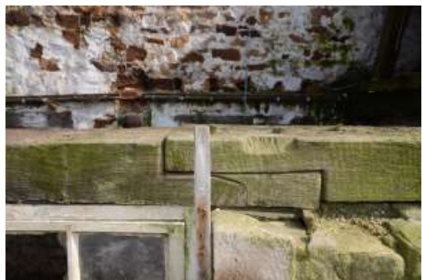
Plate 22 Wall plate towards the north end of the southwest outshut
