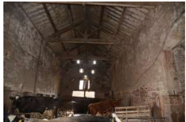
Plate 27 Interior of the barn, looking south
