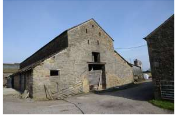
Plate 23 Southeast elevation of the barn
