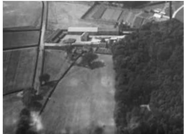
Plate 18 Aerial view of the farm, looking northwest, 1925 © Britain from Above, EPW013897
