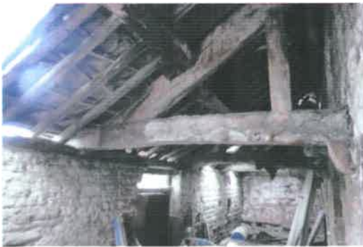
Photo 9 - Interior to south-west lean-to (southern half which is not lined).
