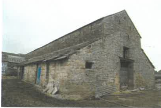
Photo 1 - View of the barn from the south, showing the south-west extension/lean-to.
