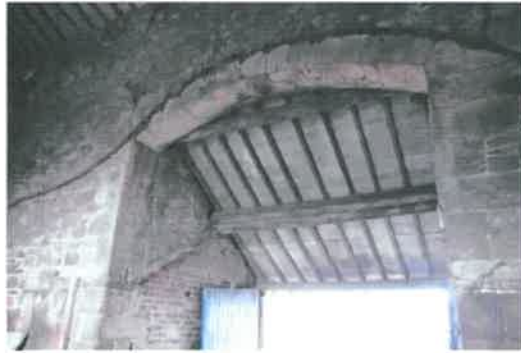
Photo 8 - Lined section of the roof leading into the main barn interior.
