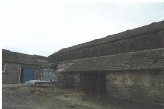
Photo 5 - South-west lean-to, showing dismantled roof section.
