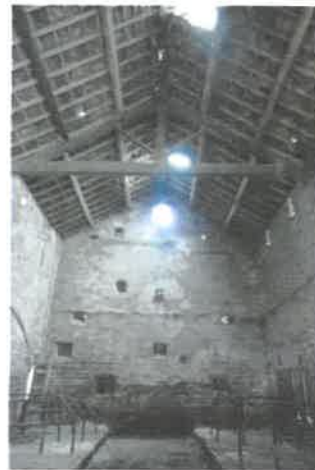
Photo 4 - Interior and roof structure to the main barn.
