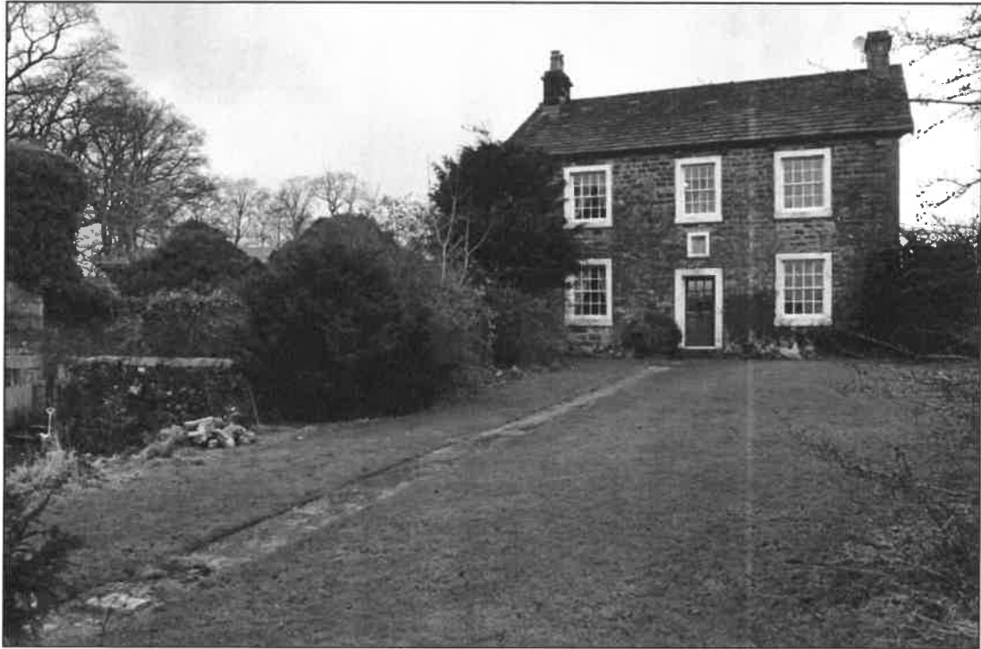
Photo 1: Farmhouse, and site of proposed extension to left
