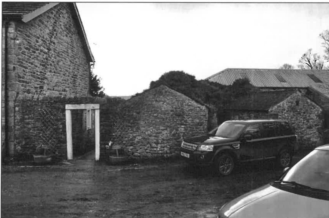
Photo 4: Rear view of domestic (left) and agricultural (right) outbuildings, to be incorporated within proposed extension
