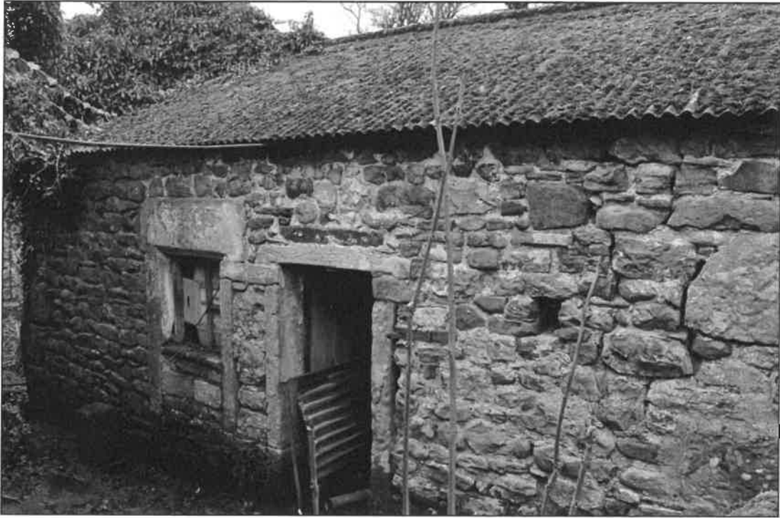
Photo 5: Agricultural outbuilding to be incorporated within proposed extension (re-used, dated lintel over left-hand doorway)
