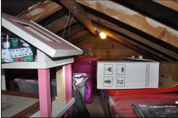
View of roof void showing shallow, cluttered space (lhs) and modern roof membrane (rhs)
