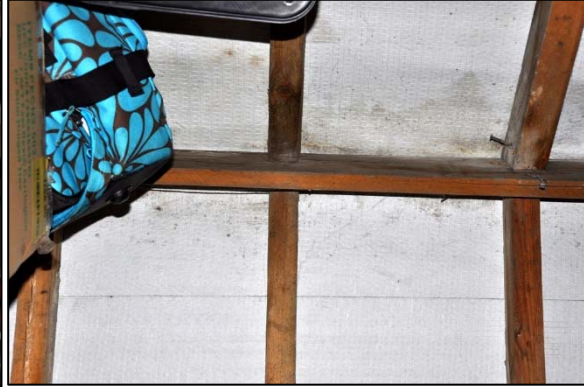
View of roof void showing shallow, cluttered space (lhs) and modern roof membrane (rhs)
