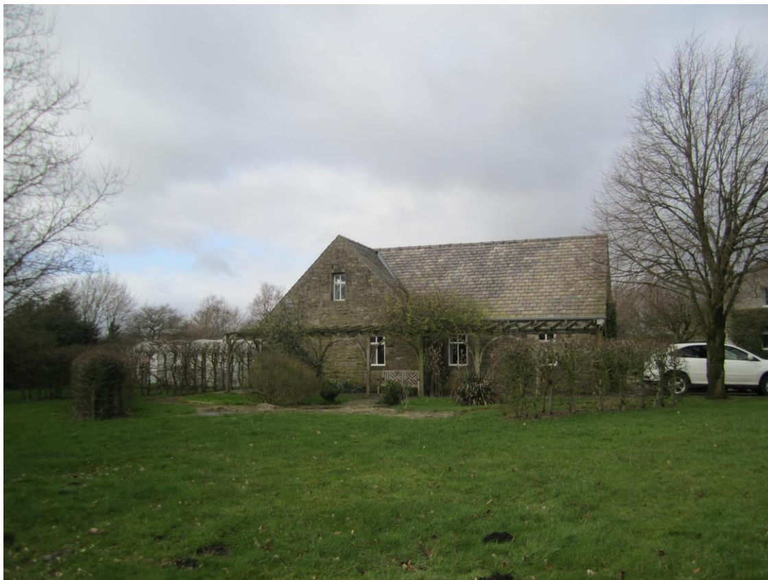
3 The southern elevation of the outbuilding. The pergola is part of a mature planting scheme.
