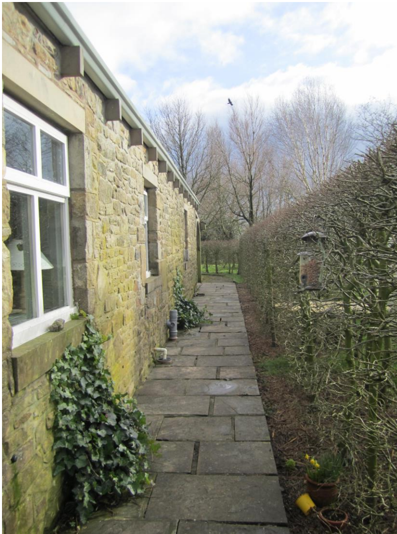
6. Western elevation well screened by hedging.
