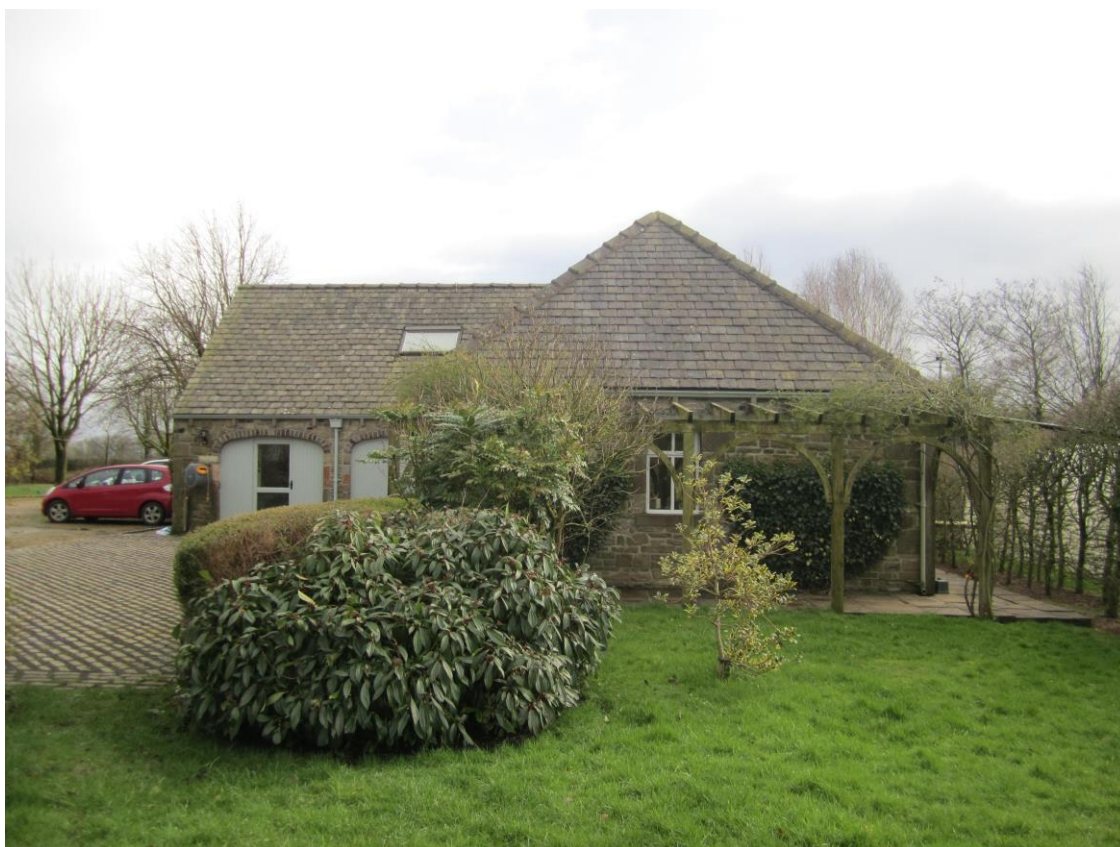
4 The northern elevation of the outbuilding. The pergola is a similar height to the adjacent beech hedge.
