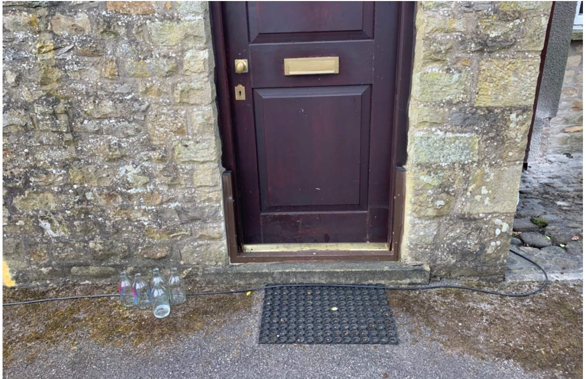
House flood barrier, installed by previous owner
