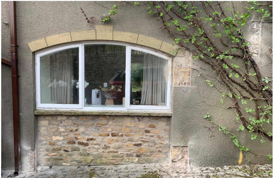
Random stone to right hand of 'wagon door', left side is blockwork and arch is decorative Art stone, bearing onto blockwork.
