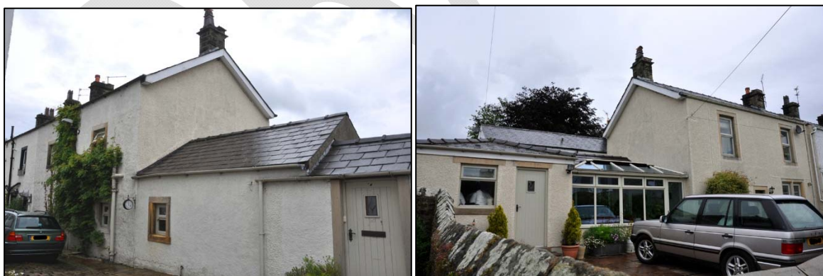
Front (lhs) and rear (rhs) elevations of 90 Regent Street showing two storey building with adjoining single storey extensions
