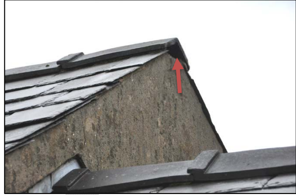
West gable of two storey section (lhs) showing tight fitting soffits with house martin nesting signs below (shown by red arrows) and west gable of single storey section (rhs) showing gap at apex with potential for use by nesting birds.
