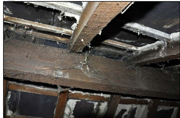
View of roof void showing no roof liner and deep rock wool (lhs) and close up view of heavy cobwebs, suggesting lack of use/disturbance (rhs)
