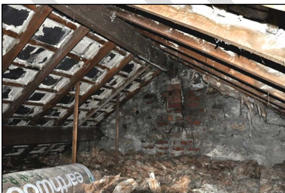
View of roof void showing no roof liner and deep rock wool (lhs) and close up view of heavy cobwebs, suggesting lack of use/disturbance (rhs)
