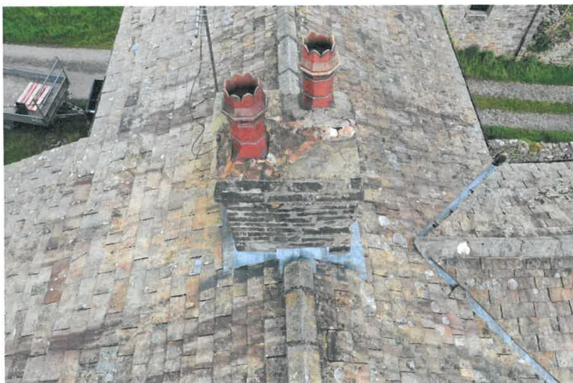
Photo 17: Close up of Chimney 1
