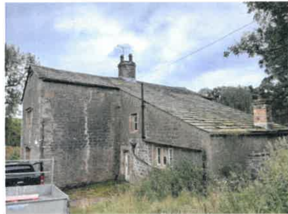
Photograph 2: View south, showing the catslide roof towards the north-west of Fooden Hall.
