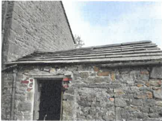
Photograph 11: North-western elevation of the outbuilding.
