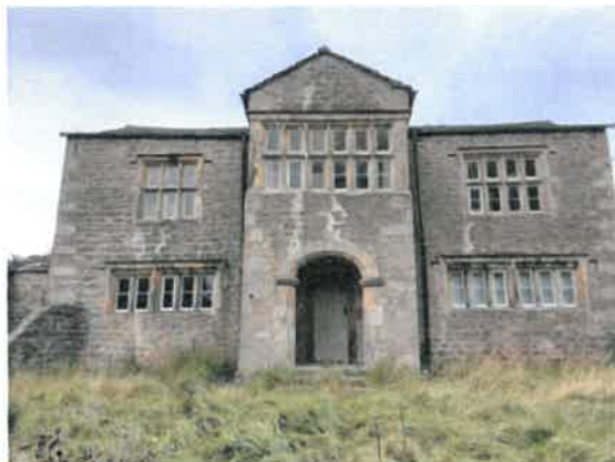
Photograph 1: South-east elevation of Fooden Hall.
