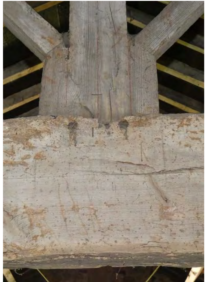
Plate 54 (left): 'II' marked on the south-west face of the north-east truss in F1
