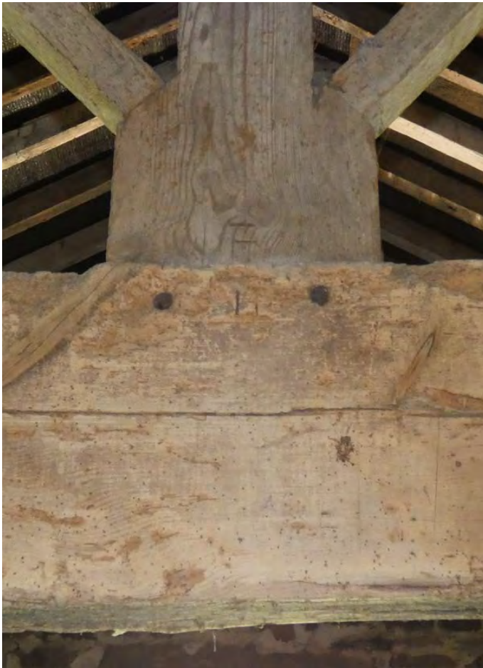
Plate 54 (left): 'II' marked on the south-west face of the north-east truss in F1
