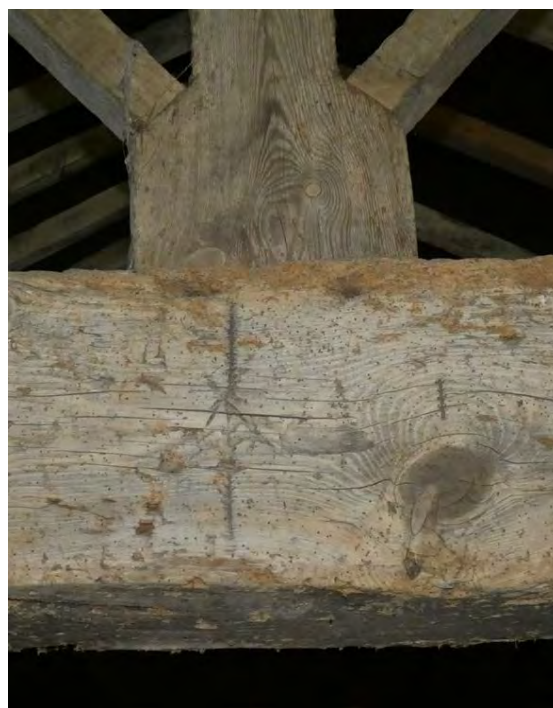
Plate 52 (left): '742' marked on the north-east face of the north-east truss in F1
