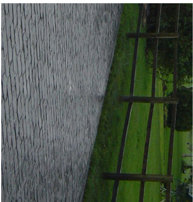
Image of imprinted concrete with cobble effect
