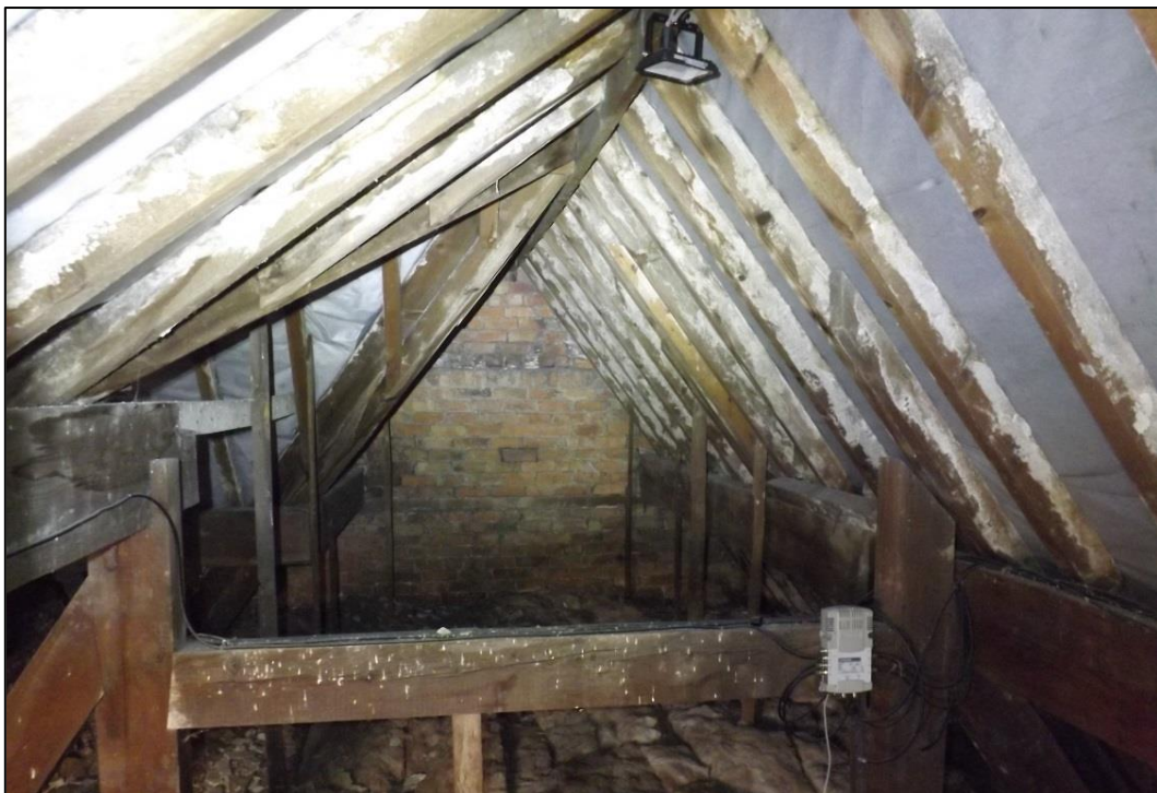
Plate 7: The loft was fully accessible and unaffected by the ongoing renovation works.
