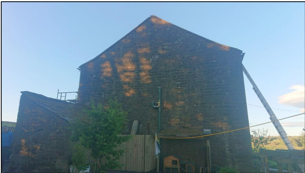
Figure 9. Gable end wall of main building showing how outbuildings are adjoined.
