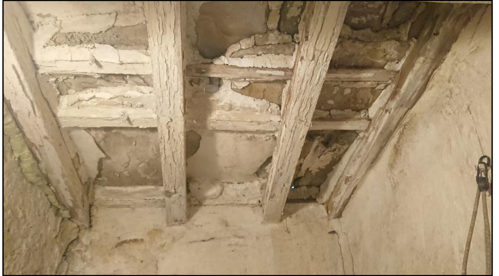
Figure 10. Roof construction within outbuilding.
