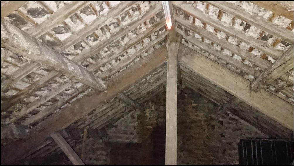
Figure 21. Roof structure internally in main building.
