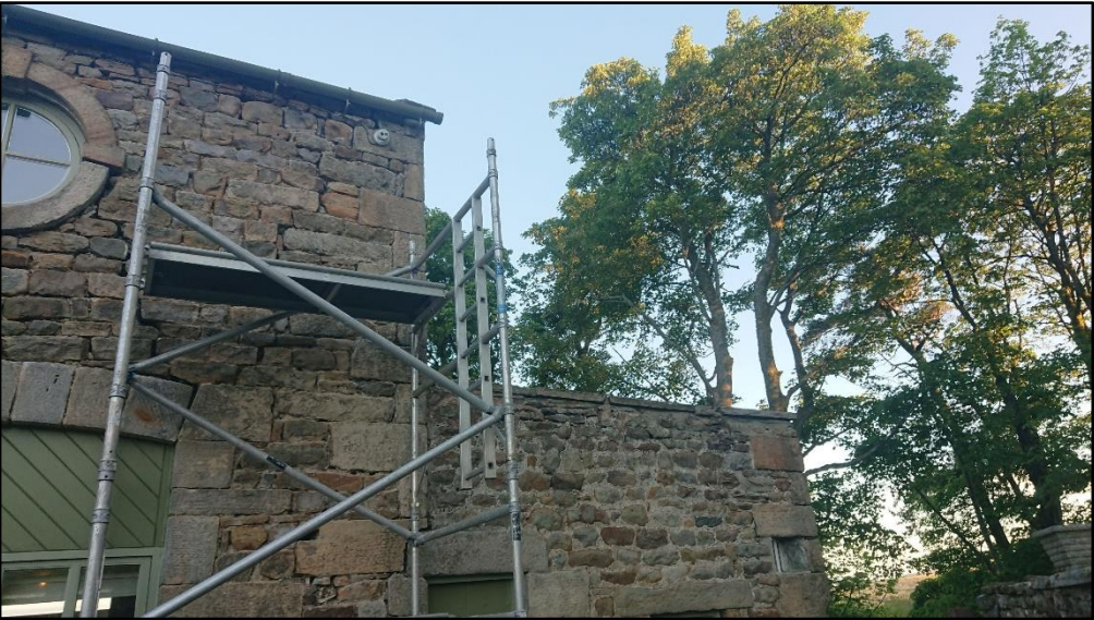
Figure 15. Close-up showing where the main building and outbuildings are adjoined.
