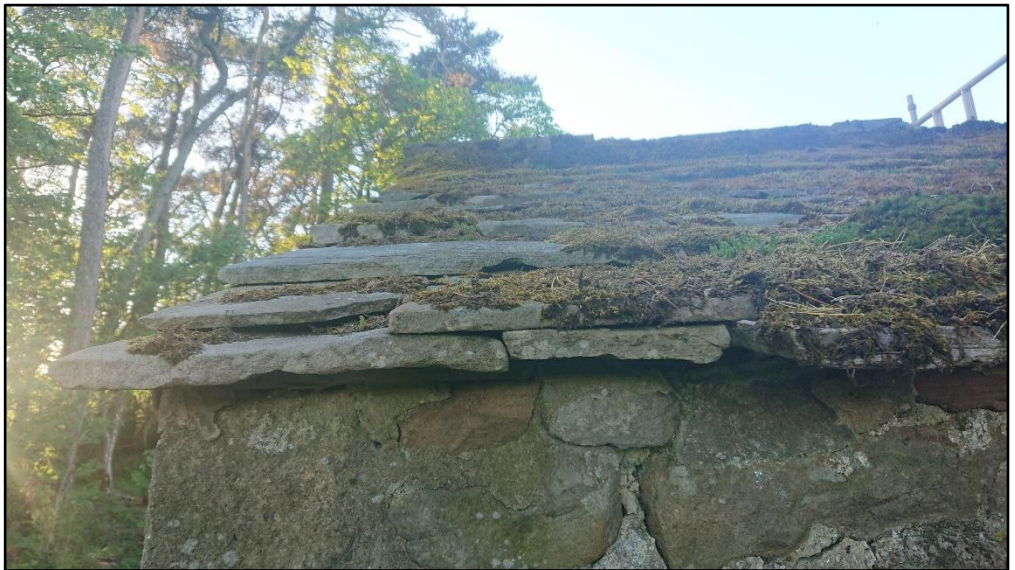
Figure 6. Roof of outbuildings close-up.
