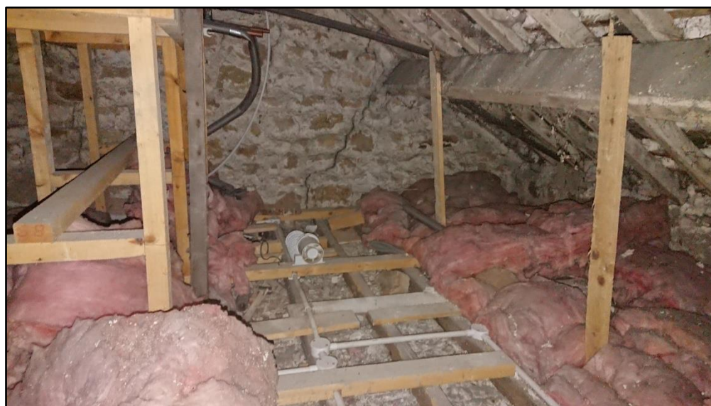
Figure 17. Loft void in main building.
