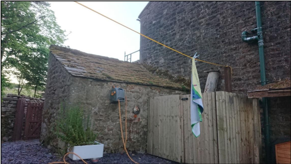
Figure 5. Rear (southern) and side (western) elevations of outbuildings.
