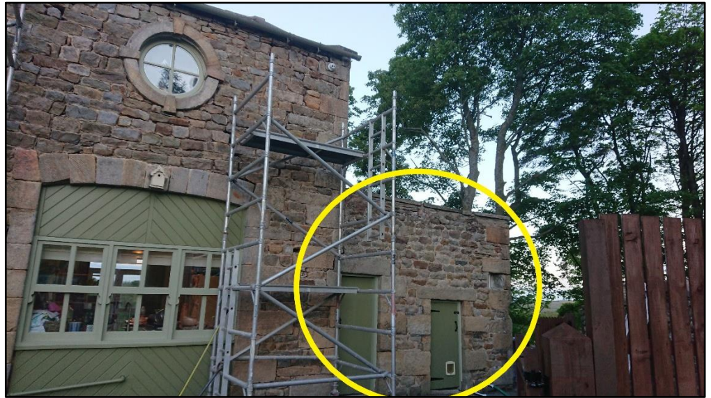
Figure 4. Front (northern) elevation of outbuildings.
