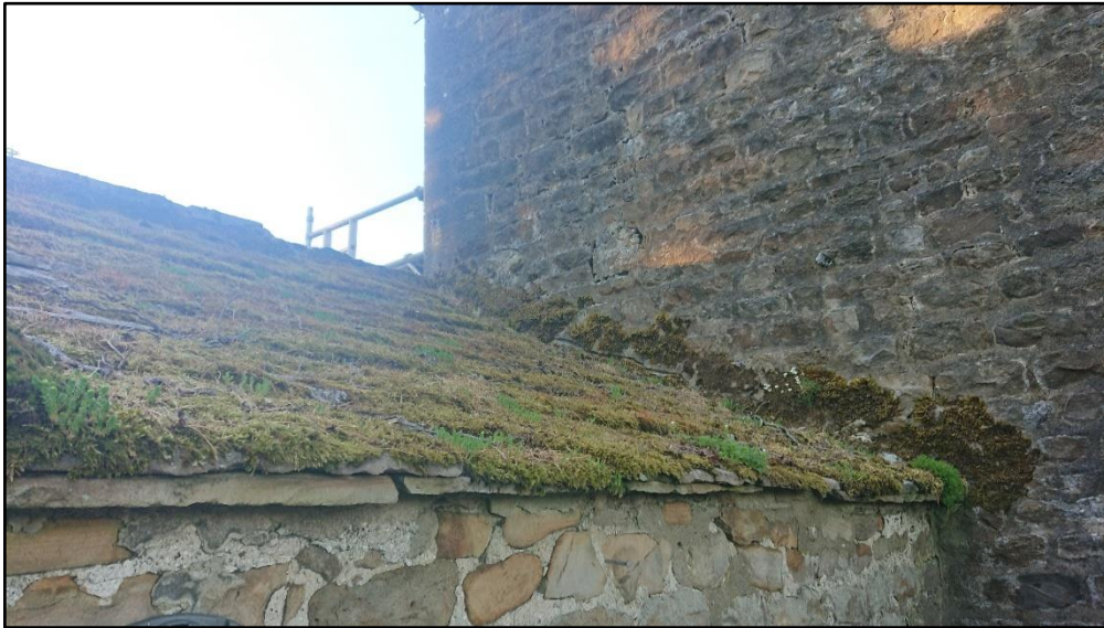
Figure 7. Roof of outbuilding.
