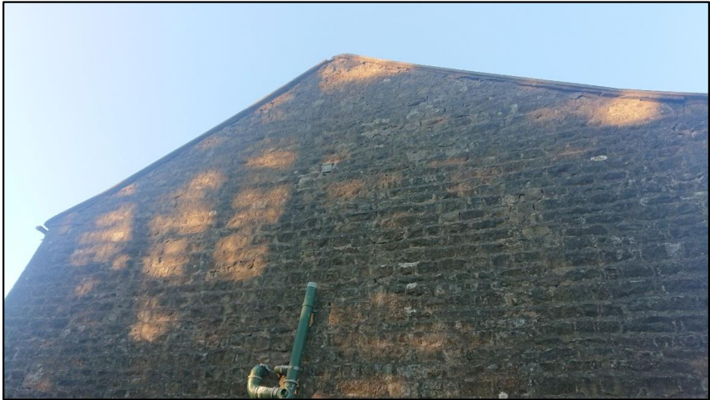
Figure 14. Western gable end wall of main building.
