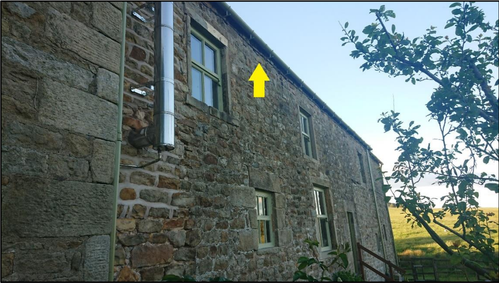
Figure 13. Rear elevation of main building with roost entrance marked.
