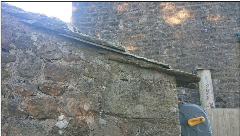
Figure 8. Outbuilding wall close-up.
