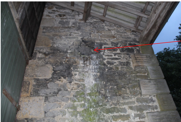
Barn Owl roost in hole in wall nest to box entrance
