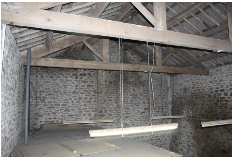
Very well sealed internal walls and wall tops
