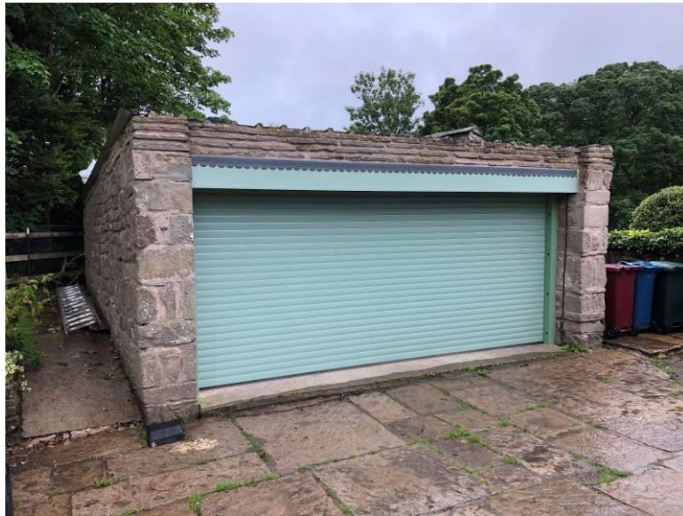
Plate 7: A view of the garage
