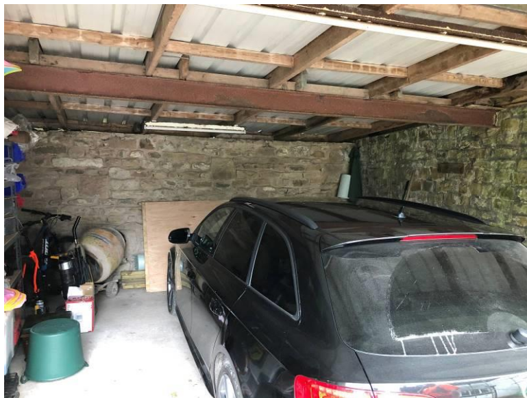
Plate 8: A view of the interior of the garage, open to the corrugated metal roof
