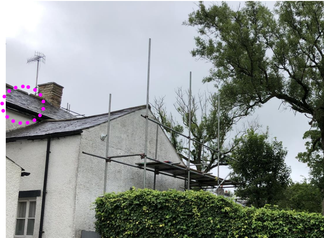
Figure 4 - Visual Aid – Suspected emergence location at roof plate level on the north-west corner of the building from which three Natterer's bats emerged during the second survey
