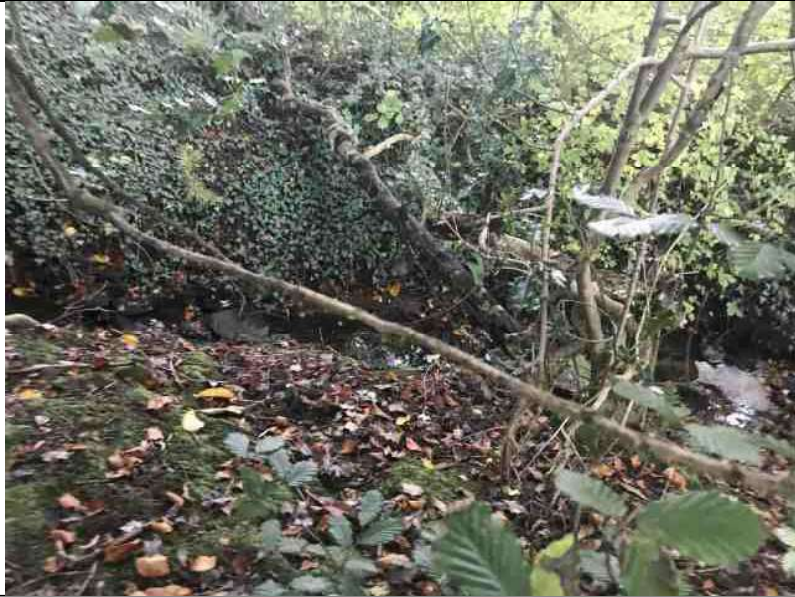
Photograph 13 (facing NE): A drain running between the site and Moor Lane at few meters below the site levels.
