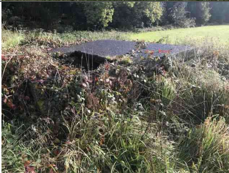
Photograph 9 (facing SE): Manhole cover adjacent to the lodge.
