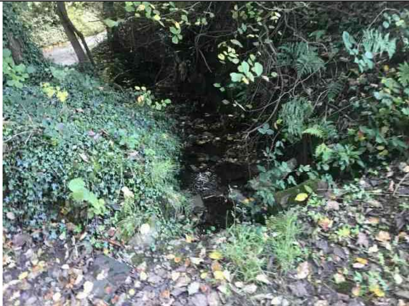
Photograph 14 (facing SE): Drain crossing beneath the site entrance.
