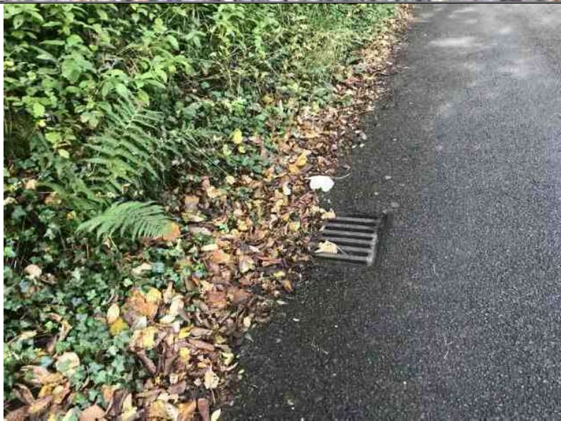
Photograph 15 (facing NW): Highway gullies in Moor Lane.
