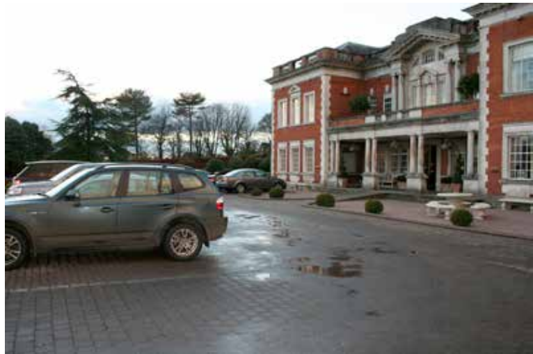
Photograph 1 The front of the hall with previous car park area
