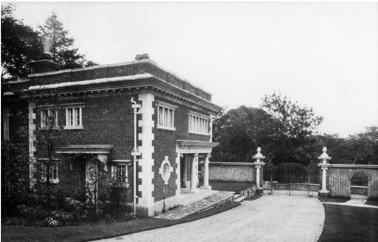
Figure 2. The lodge and gates. This photograph must also date from shortly after completion of the works. The lodge is unchanged apart from the addition of a car port and some alterations to the parapet details.
