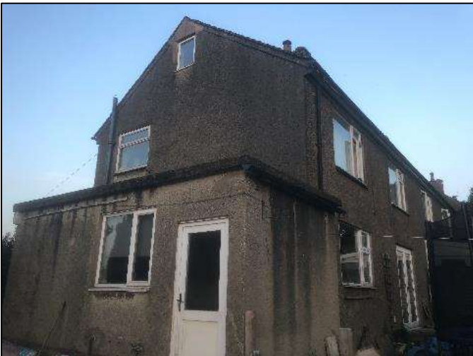
Photo 2: Single-storey extension to the gable end.
