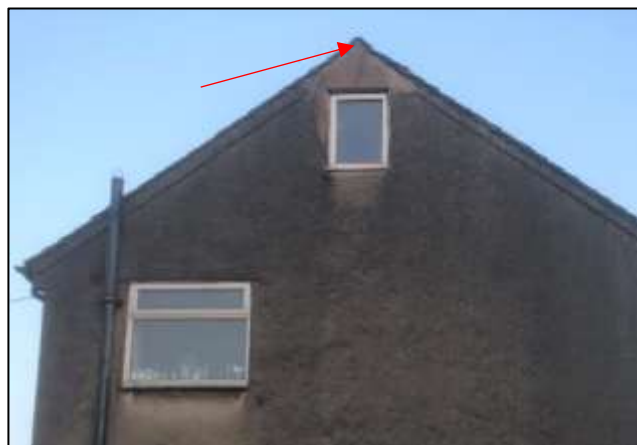
Photo 4: The gable end ridge tile with mortar gap at the uppermost point.
