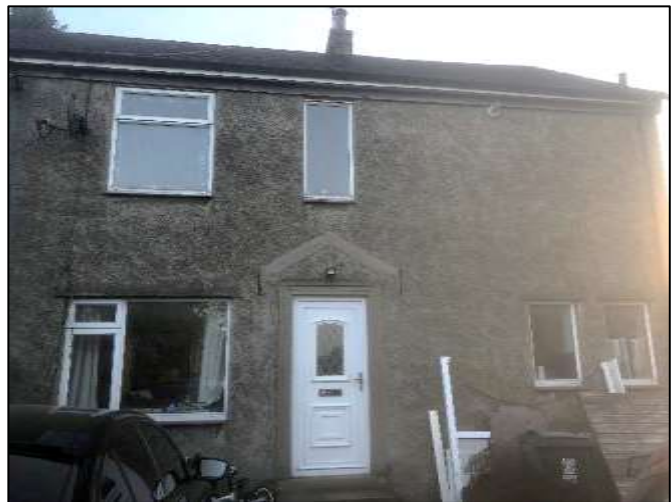
Photo 1: East facing elevation of the survey building.
