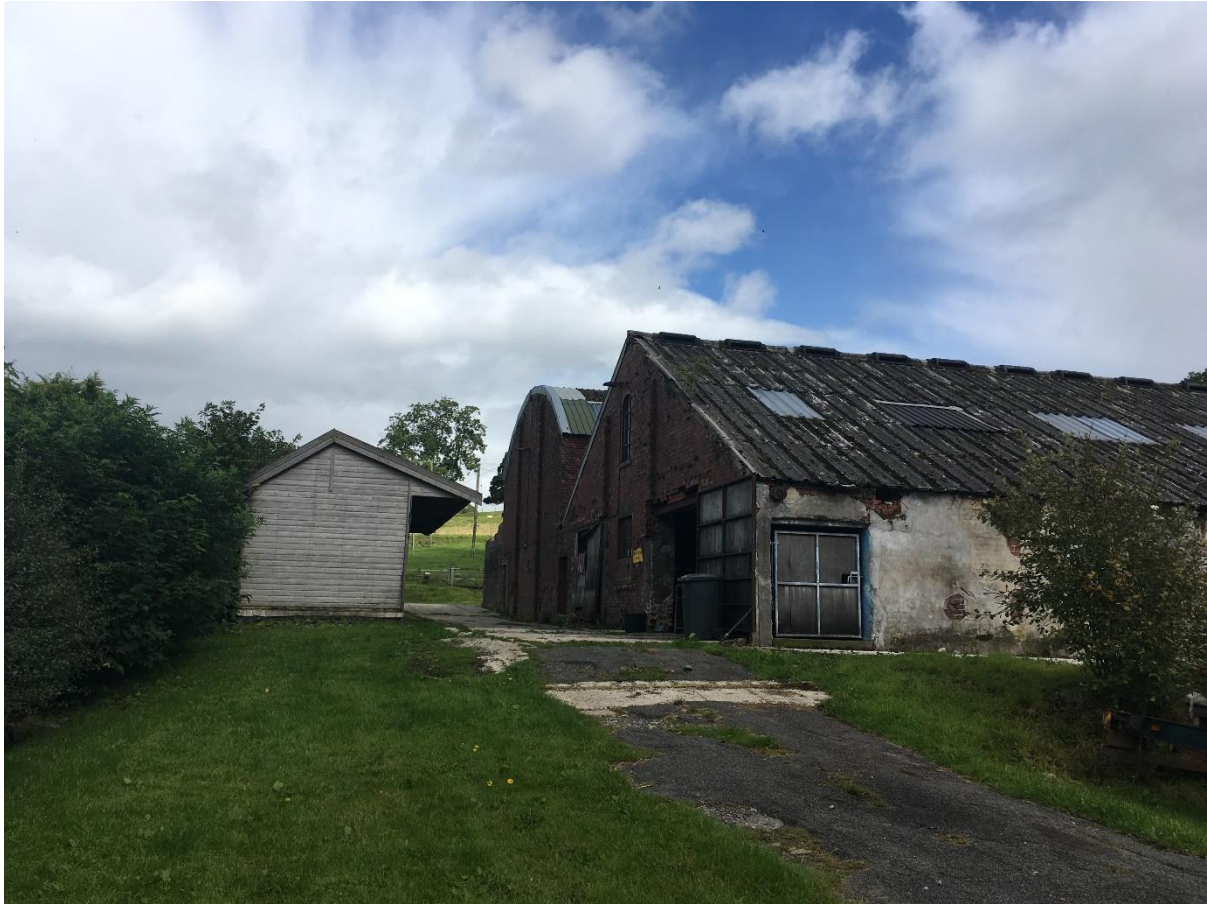
Photograph I: Proposed buildings viewed from the south
