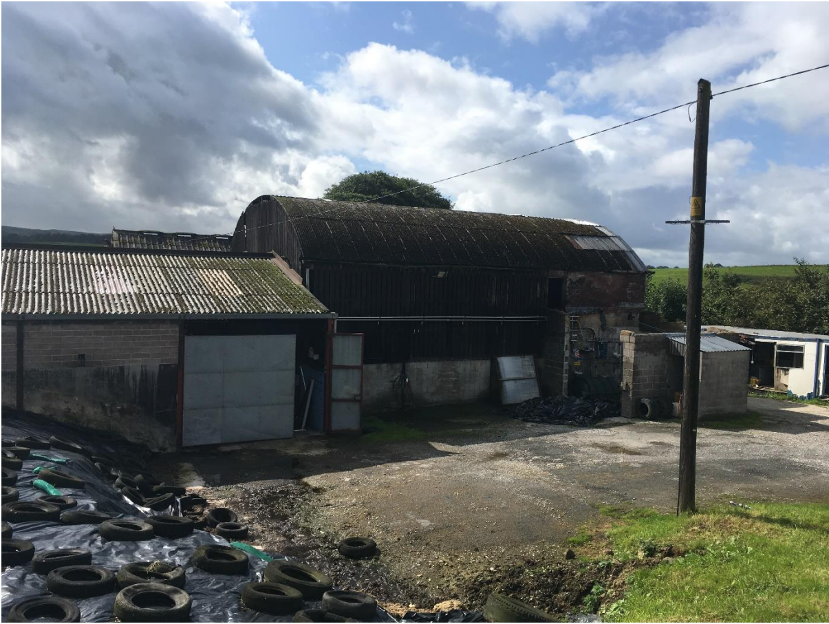
Photograph 2: Dutch Barn viewed from northeast
