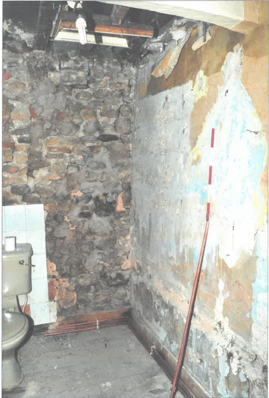
Photo 2: Location of former stairs to second floor. Now bathroom. Diagonal line in plaster immediately above red and white scale.
