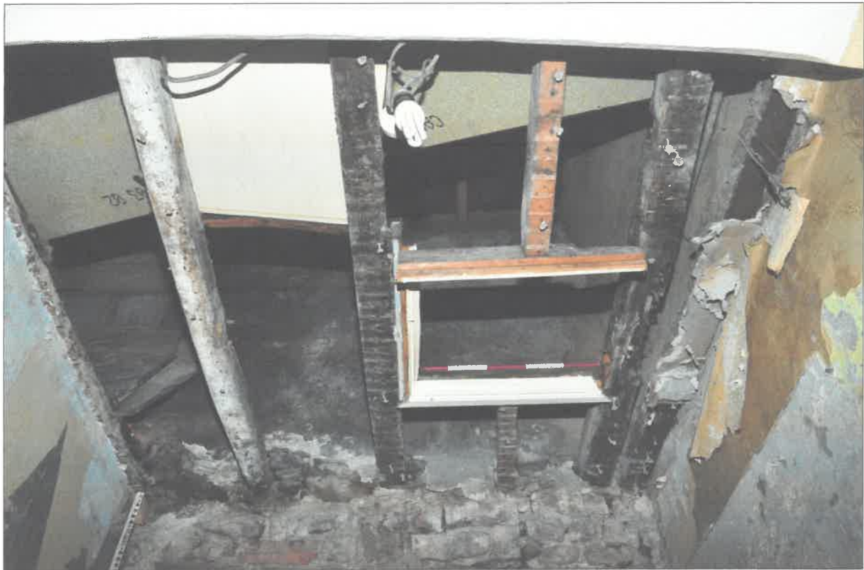
Photo 3: Modern trapdoor within infilled stairwell. Original limewashed joists at left.
