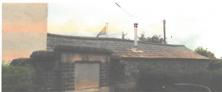
Side elevation from the adjacent public garden.
