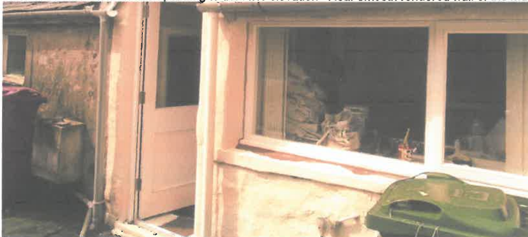
The outrigger has a slobbered render finish to the garden facing elevation, partially white painted.
