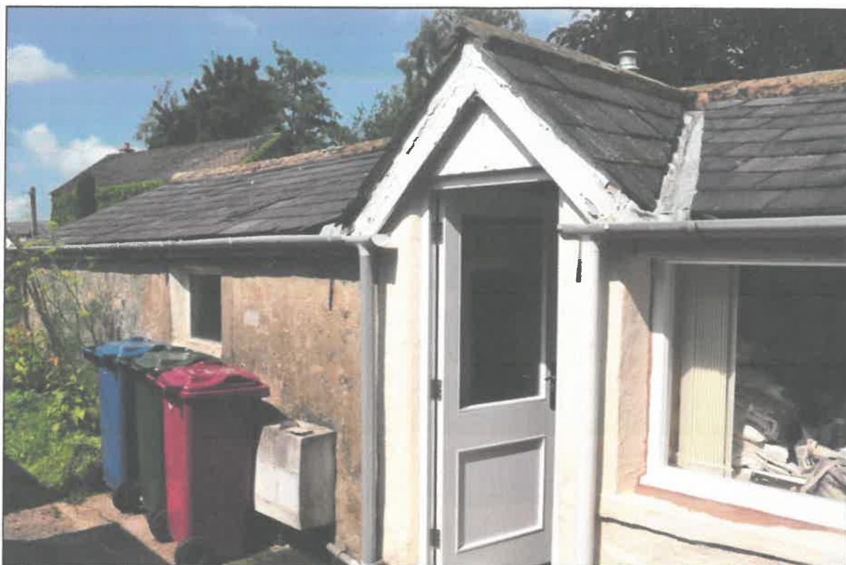
Photo 13: Rear wing (former loom-shop): south side, with altered doorway
