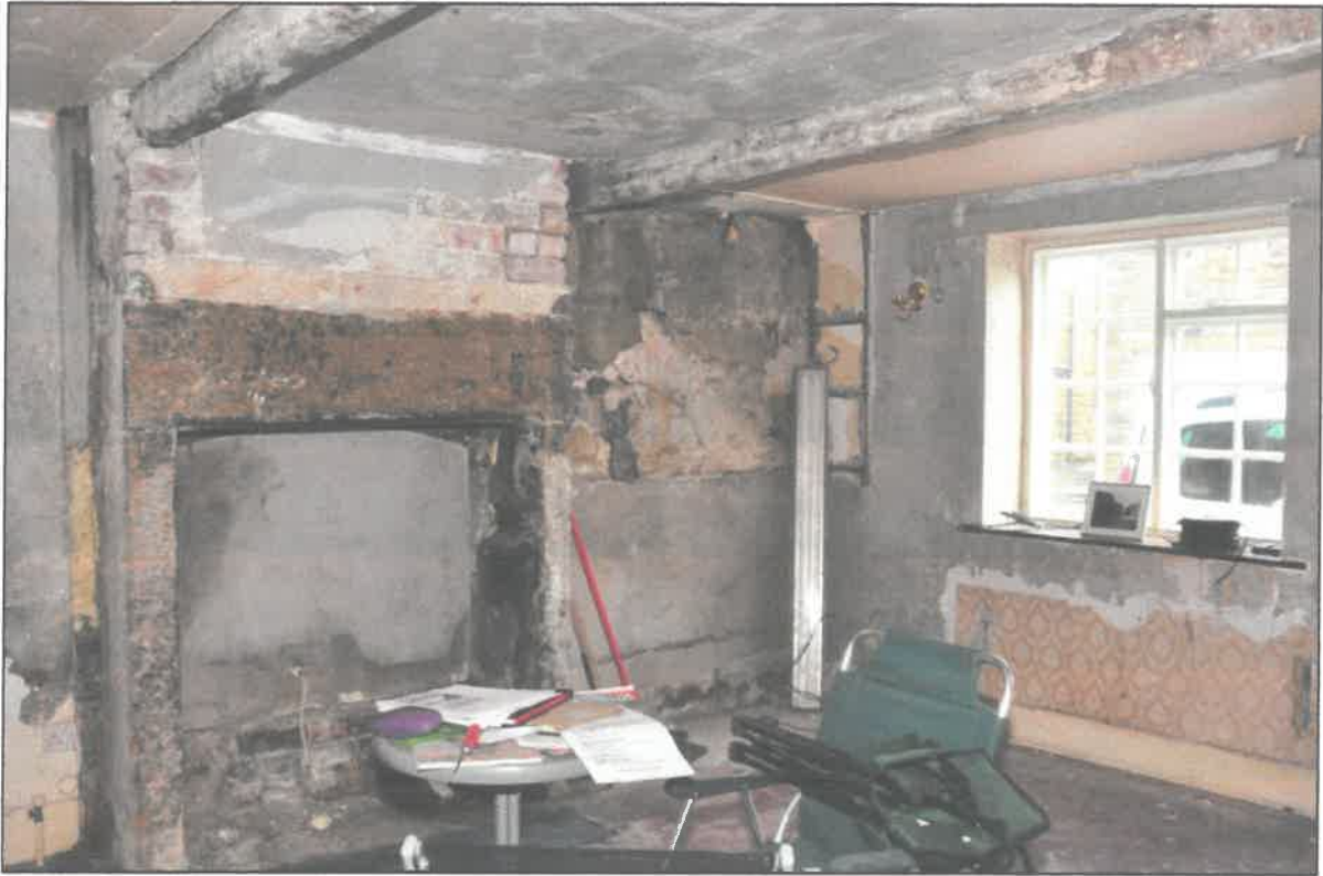
Photo 5: Front fireplace on ground floor
