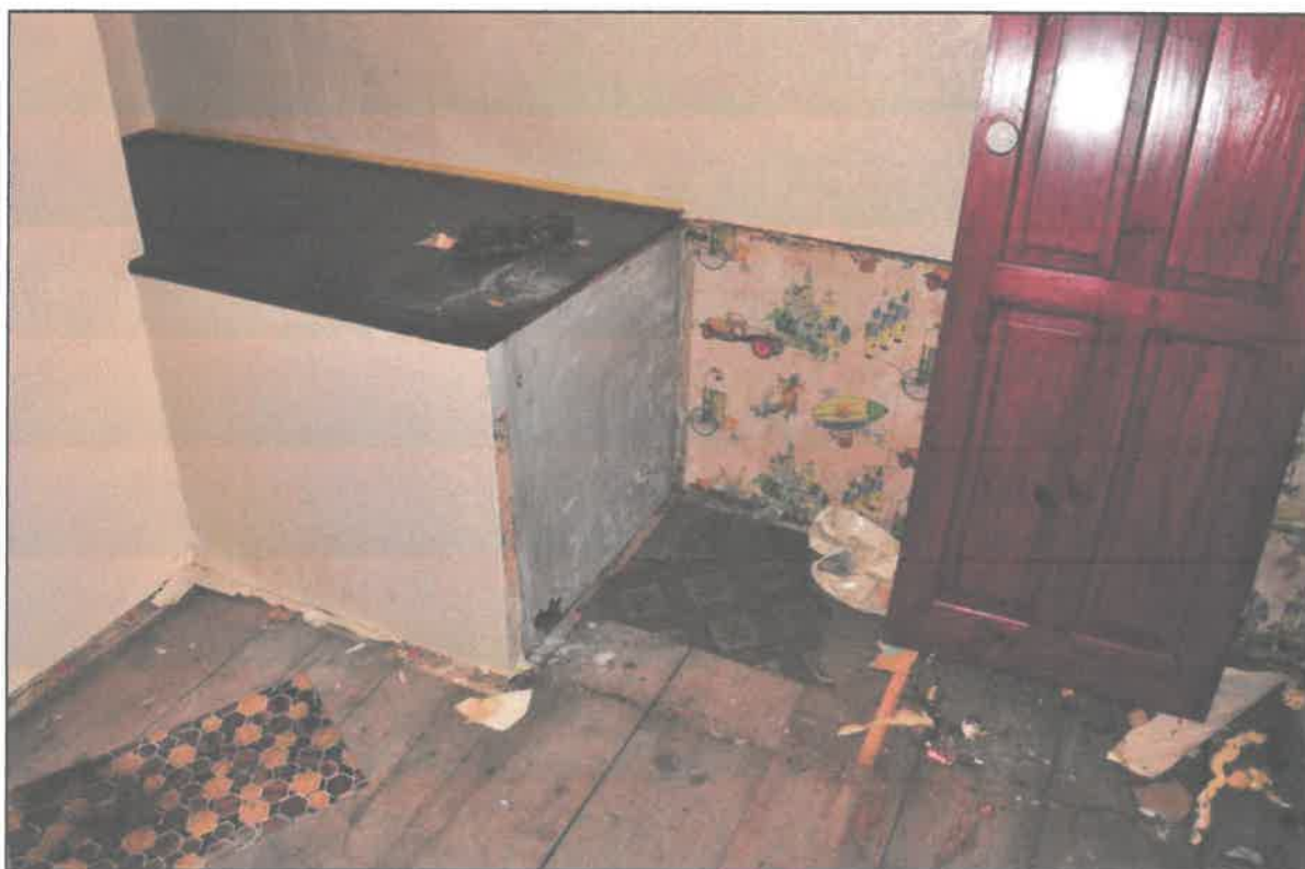
Photo 8: Site of former staircase aperture, within first floor
