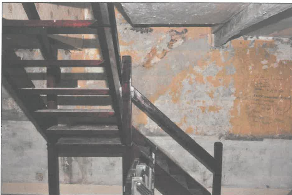
Photo 7: Present staircase, within scar of predecessor in plaster behind
