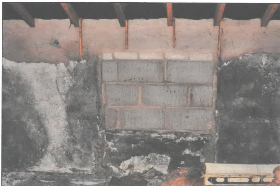
Photo 12: Blocked window, west side of second floor
