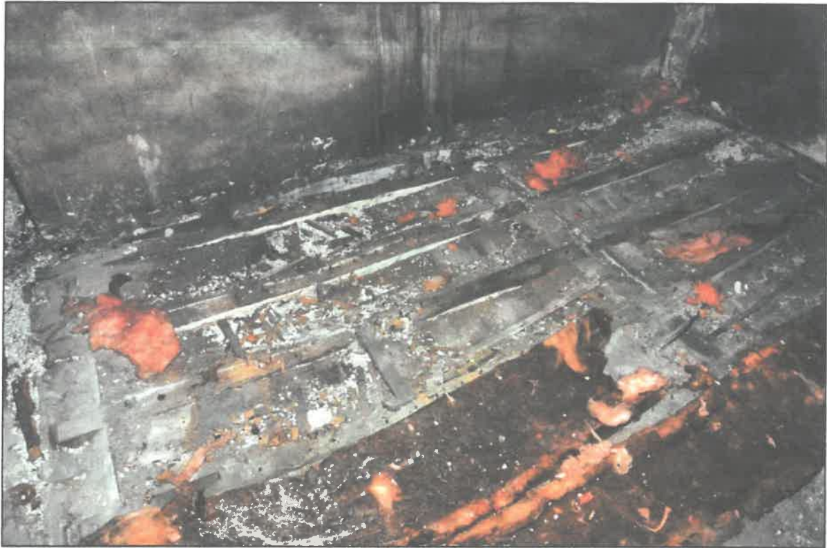
Photo 9: Upper view of joists on second floor
