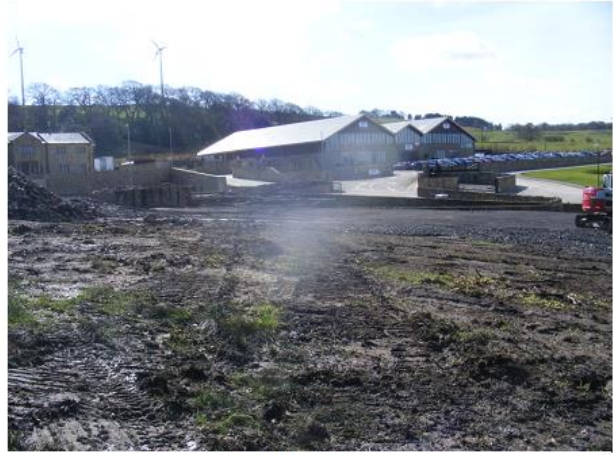
PHOTO 2 Central Area of Rough Ground.
