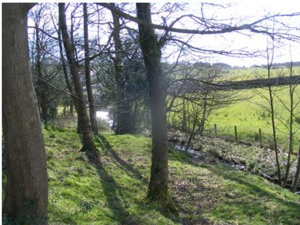
PHOTO 15 View of Northern Culvert.
