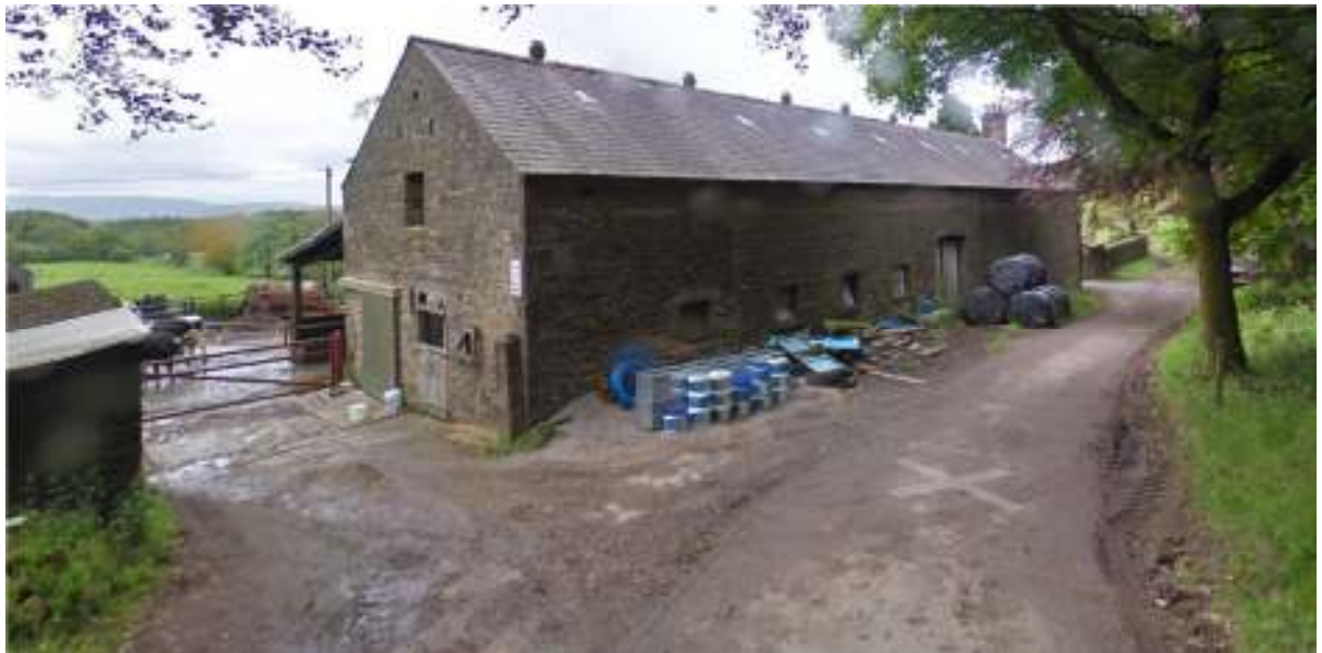
Termination of no through road – Viewed South.
