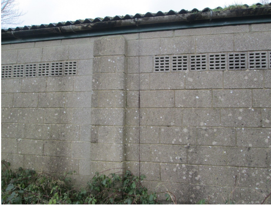
PHOTO 7 – VIEW OF MOVEMENT JOINT TO FRONT ELEVATION
