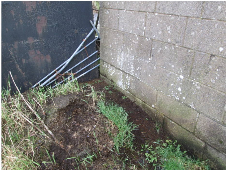
PHOTO 8 – HIGH GROUND LEVEL TO LEFT HAND END OF FRONT ELEVATION
