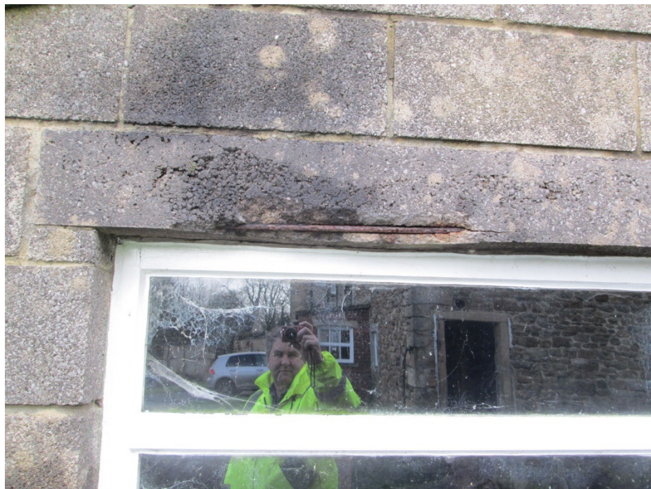
PHOTO 6 – VISIBLE REINFORCEMENT TO WINDOW LINTEL ON RIGHT HAND GABLE WALL
