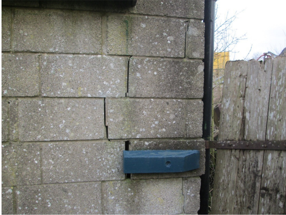
PHOTO 5 – CRACKING AND DISPLACEMENT OF BLOCKS TO RIGHT HAND SIDE OF RIGHT-HAND GABLE WALL
