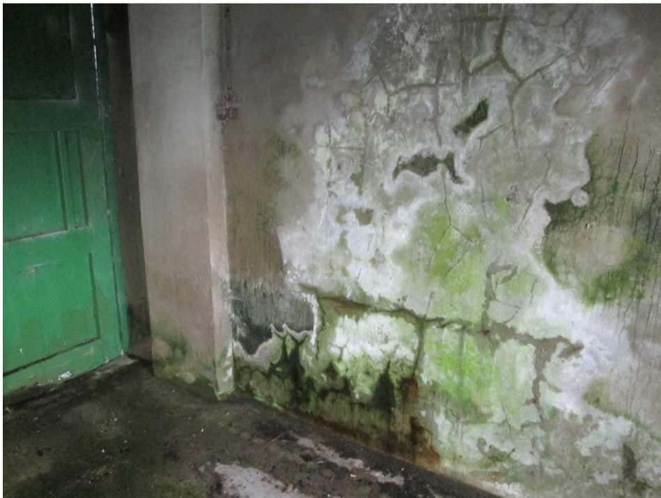
PHOTO 16 – DAMPNESS TO INNER WALL WITHIN STORE
