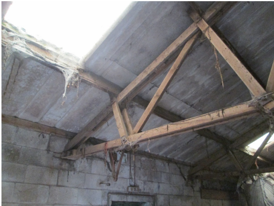
PHOTO 12 – VIEW OF TRUSS SITTING ON INNER LEAF
