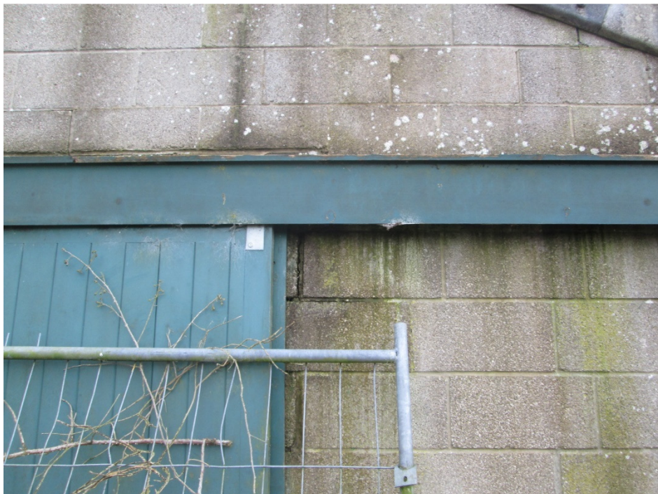
PHOTO 10 – CRACKING ABOVE LINTEL AND BELOW DOOR RUNNER TO LEFT HAND GABLE
