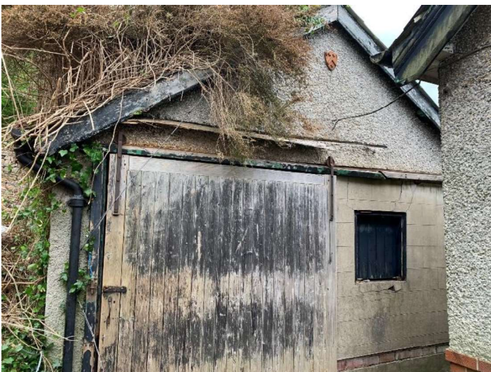
Figure 6, Garage/workshop (Authors Own, 2020)
