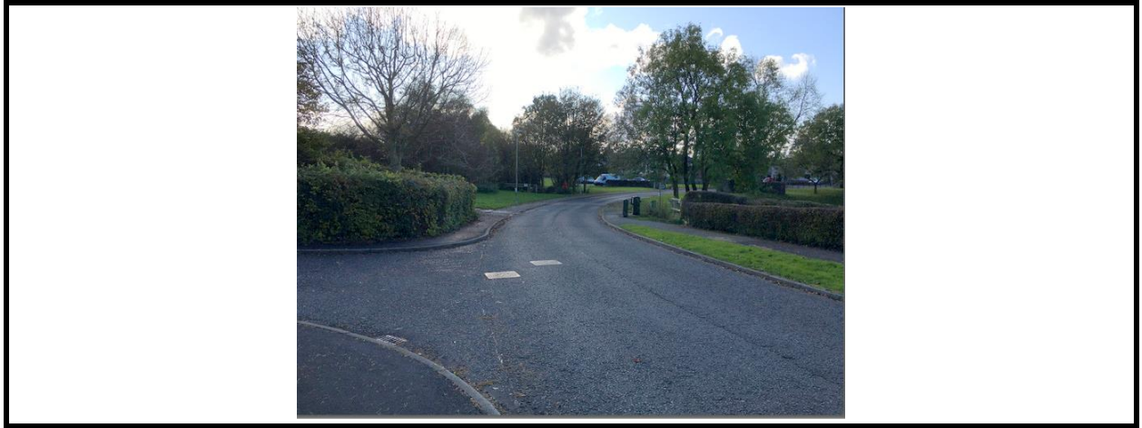
View to site access from eastside
