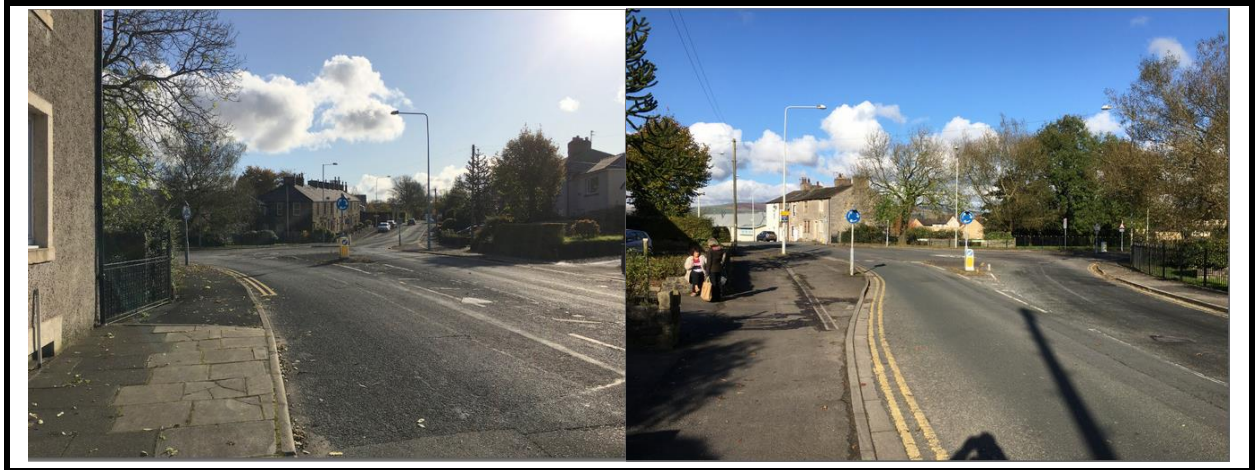
View along Pendle Road south and north to Highmoor Park junction
