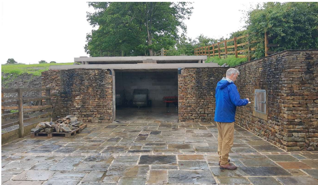
Figure 2 Agricultural Store South East facade
