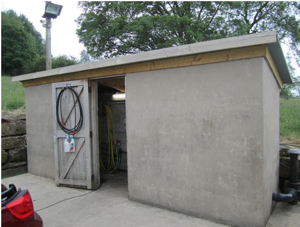
4 Existing car valeting cabin.
