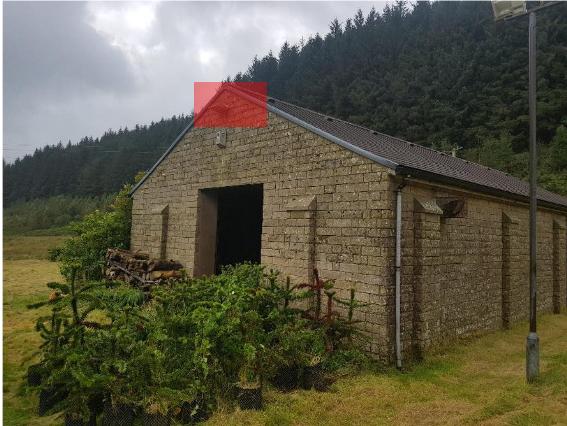
Image 1. Eastern elevation with bat emergence location highlighted red.
