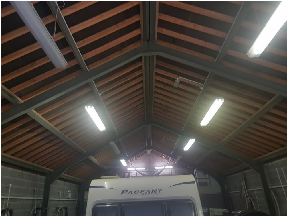
Image 4. Internal of B1 workshop/fish hatchery.
