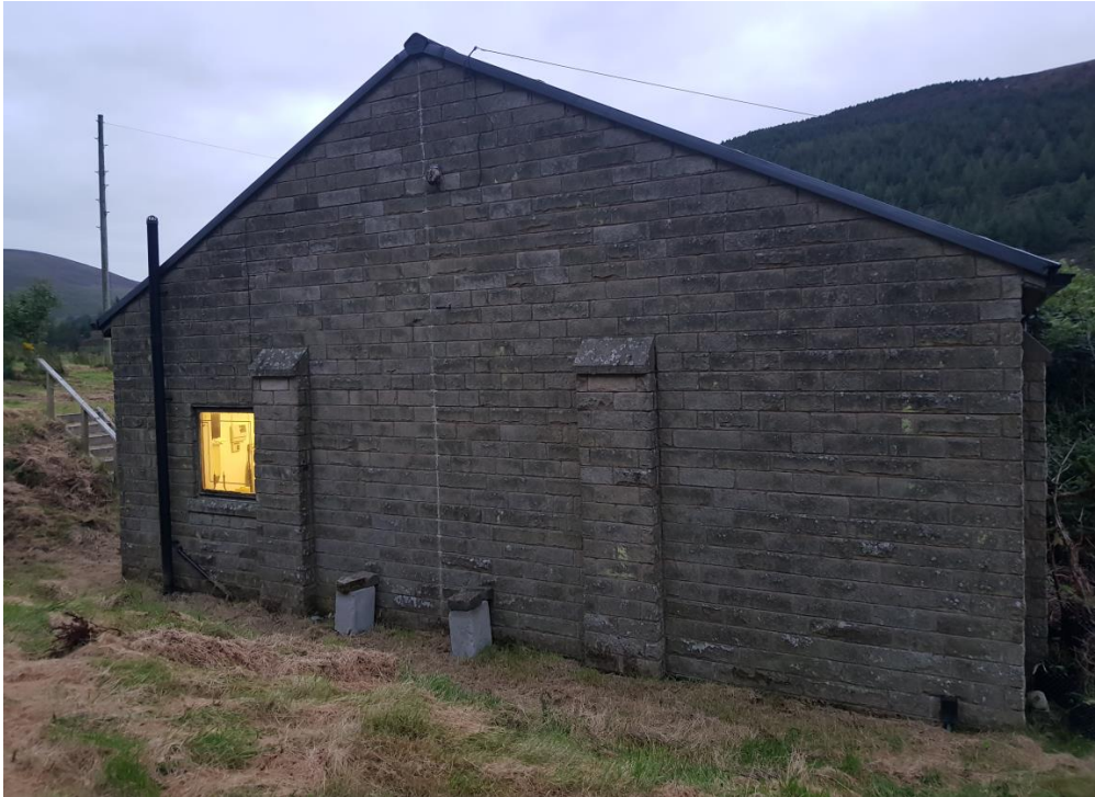
Image 3. Western elevation of B1.
