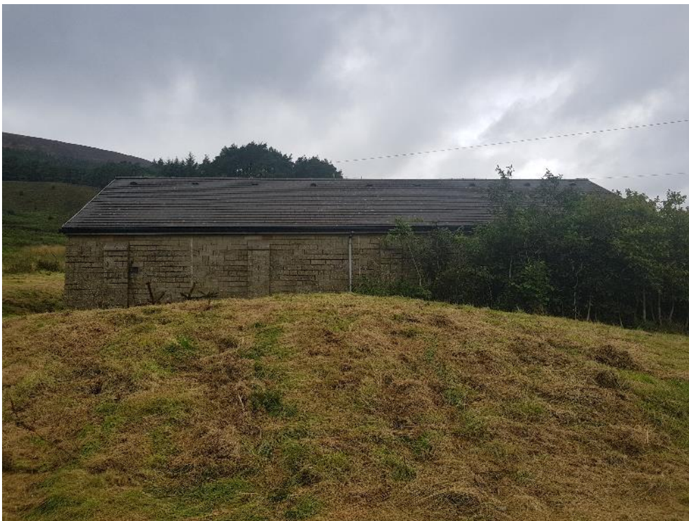
Image 2. Southern elevation of B1.
