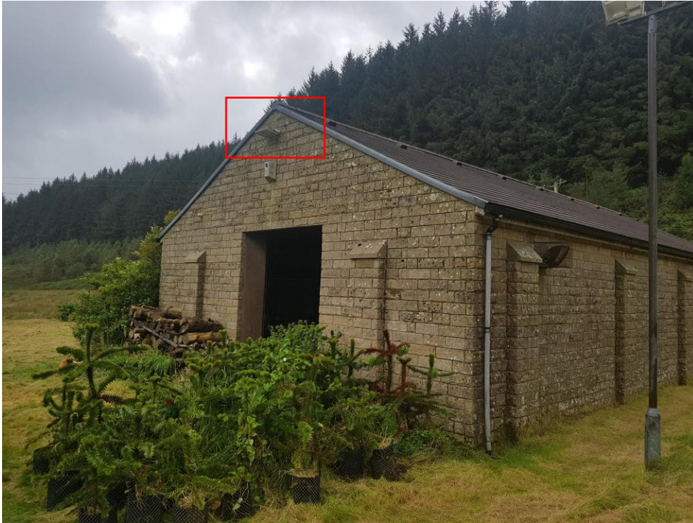
Image 1. Eastern elevation of B1 with bat emergence location highlighted red.
