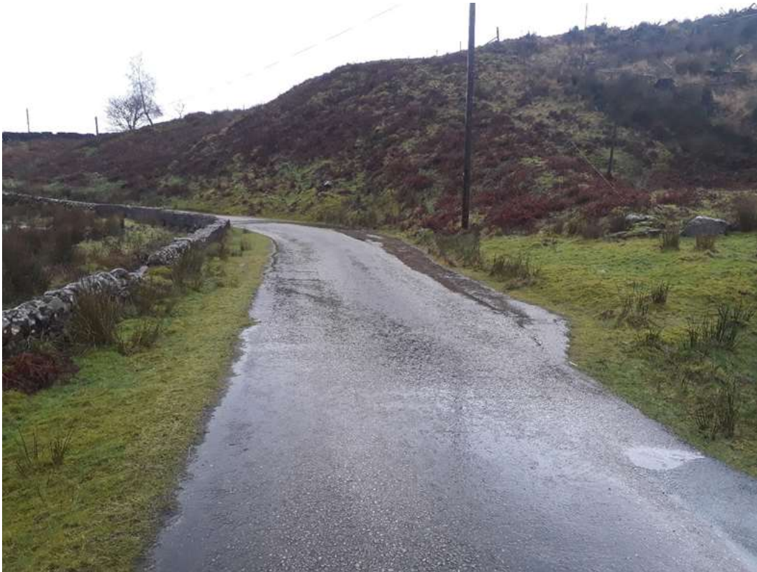
This is another passing place at the other side of the bend after pin 5
