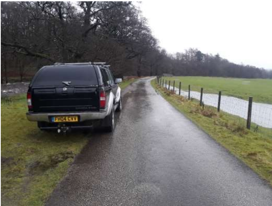
'Hard shoulder' (gravel / rock under the grass) (south of pin no.5)
