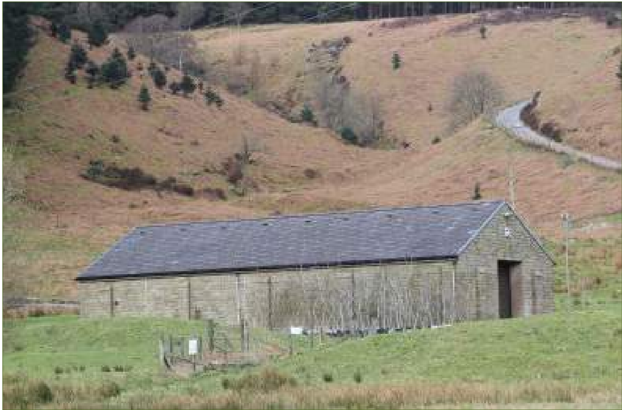
Figure 21 - View from Whitendale Road looking north towards the main fish hatchery building within the Site.
