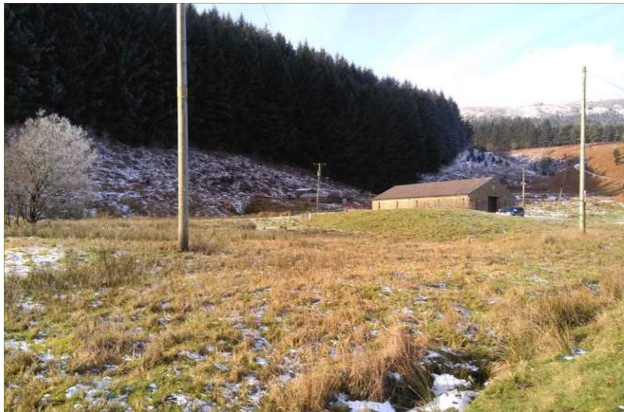
Figure 5 - View looking north-west towards the Site with plantation located to the slopes of Staple Oak Fell to the left of view.
