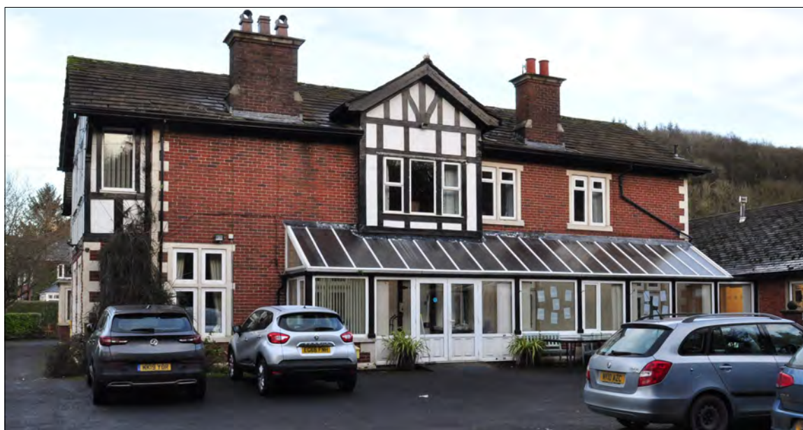
South-west elevation with sun-room proposed for replacement.
