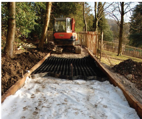
Fallbarrow Park, Windermere: CellWeb TRP® Installation
